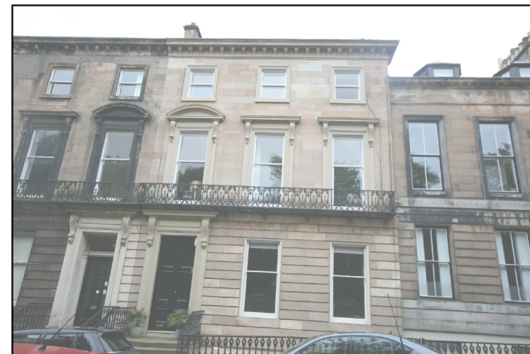
EXISTING PHOTOGRAPH OF FRONT
