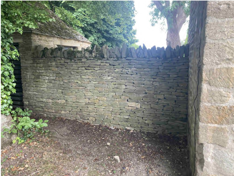
Existing wall (Garden side)
