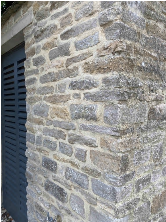
Pointed stone wall on existing plant room to be replicated
