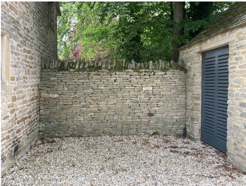
Existing wall (Drive side)
