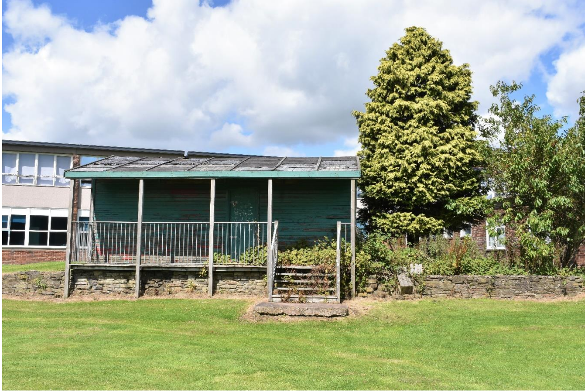
Photograph P1 – existing building front elevation
