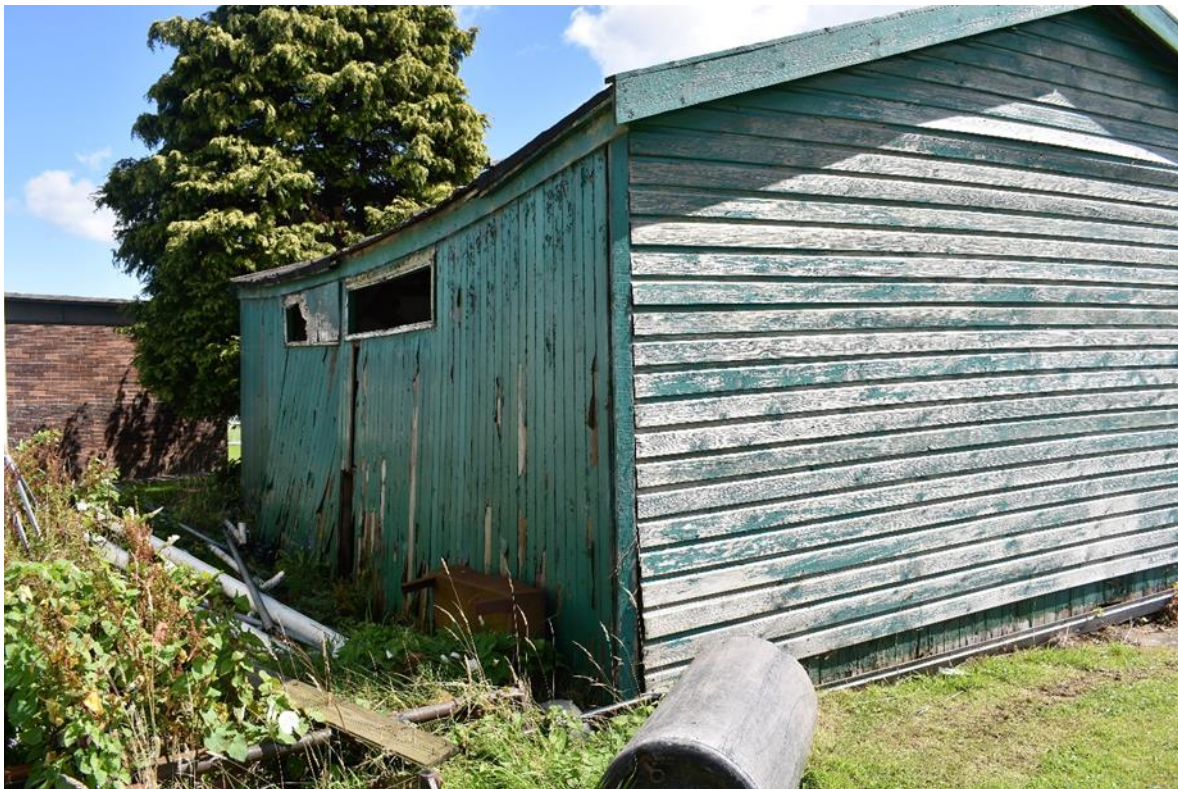
Photograph P2 – existing building rear elevation
