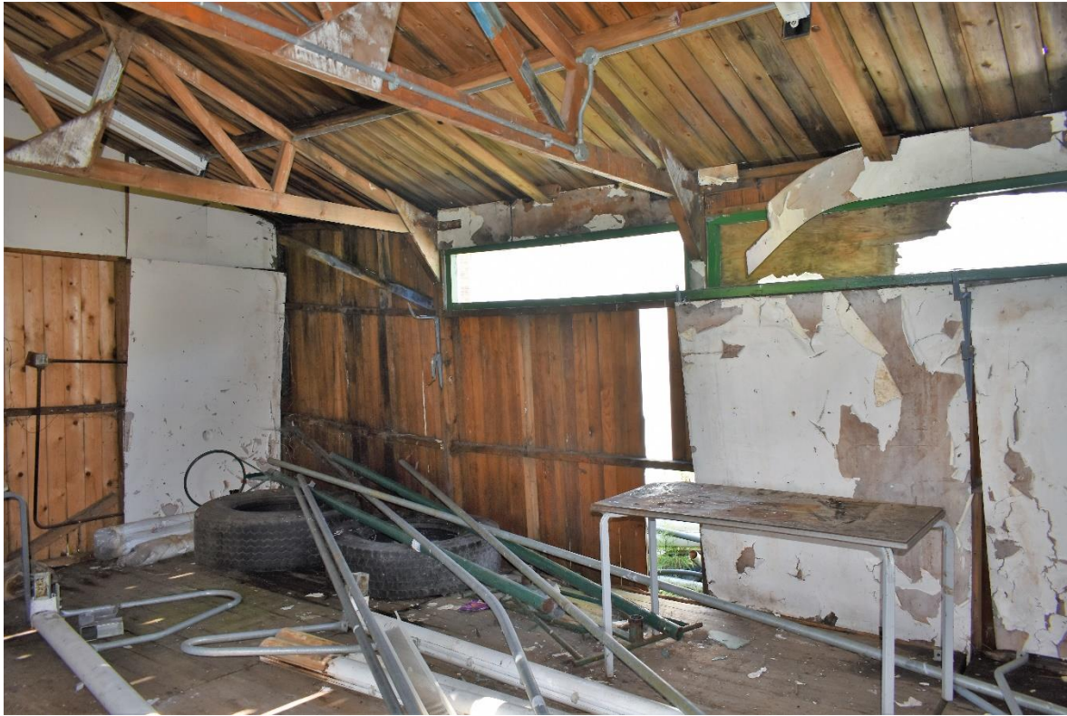
Photograph P3 – existing building internal
