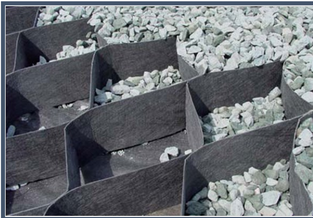
Figure 11 Examples of Cellweb filling with angular stone
