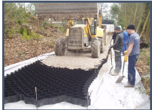
Figure 11 Examples of Cellweb filling with angular stone
