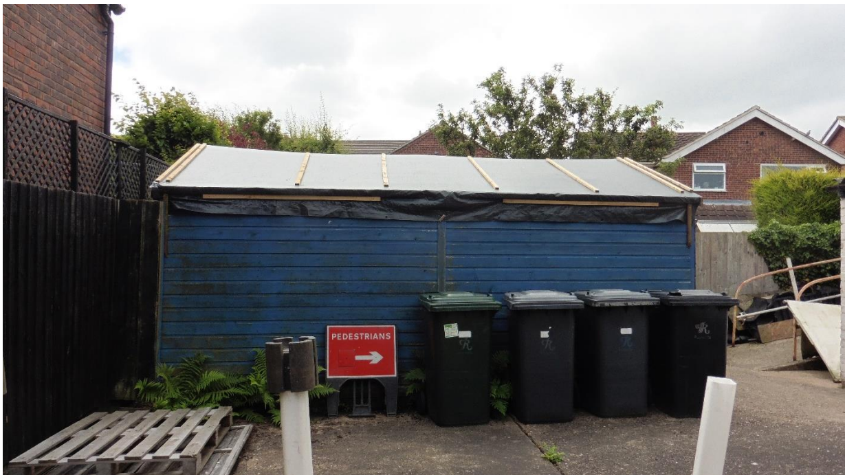
Photograph 4: The timber shed located to the south-east of the village hall.
