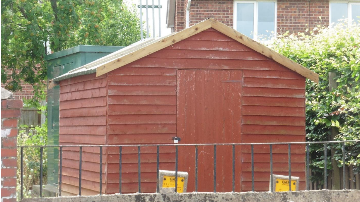
Photograph 3: The timber shed located to the west of the village hall.
