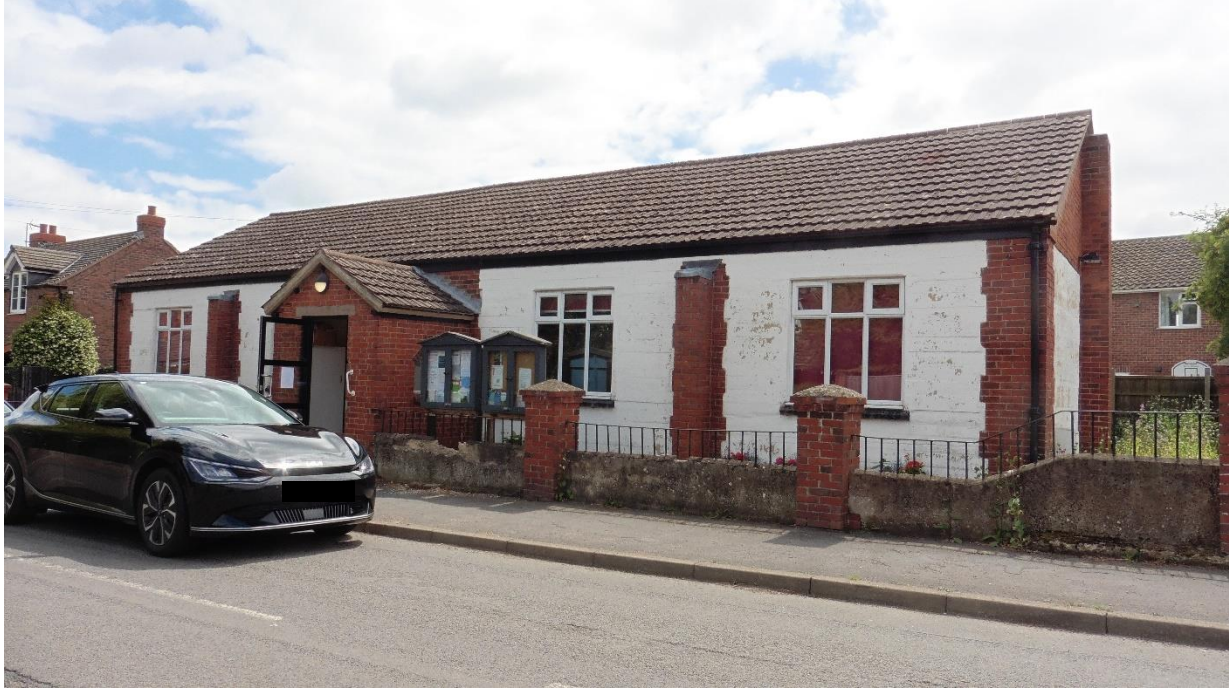
Photograph 1: Langar-cum-Barnstone Village Hall, taken from the north-west, showing the mixed construction of brick and painted ironstone and the porch attached on the northern elevation.
