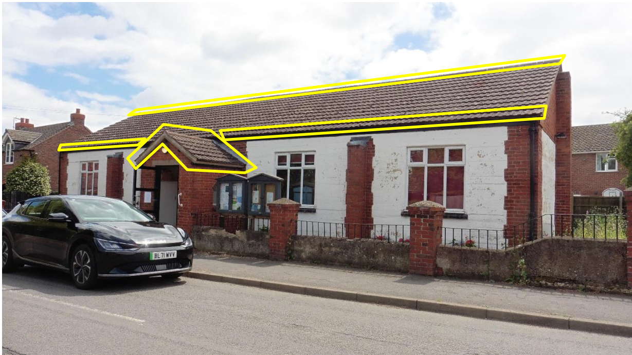
Figure 2 - showing the areas that must be soft stripped by hand in advance of demolition, under the supervision of a bat ecologist (areas highlighted in yellow).
