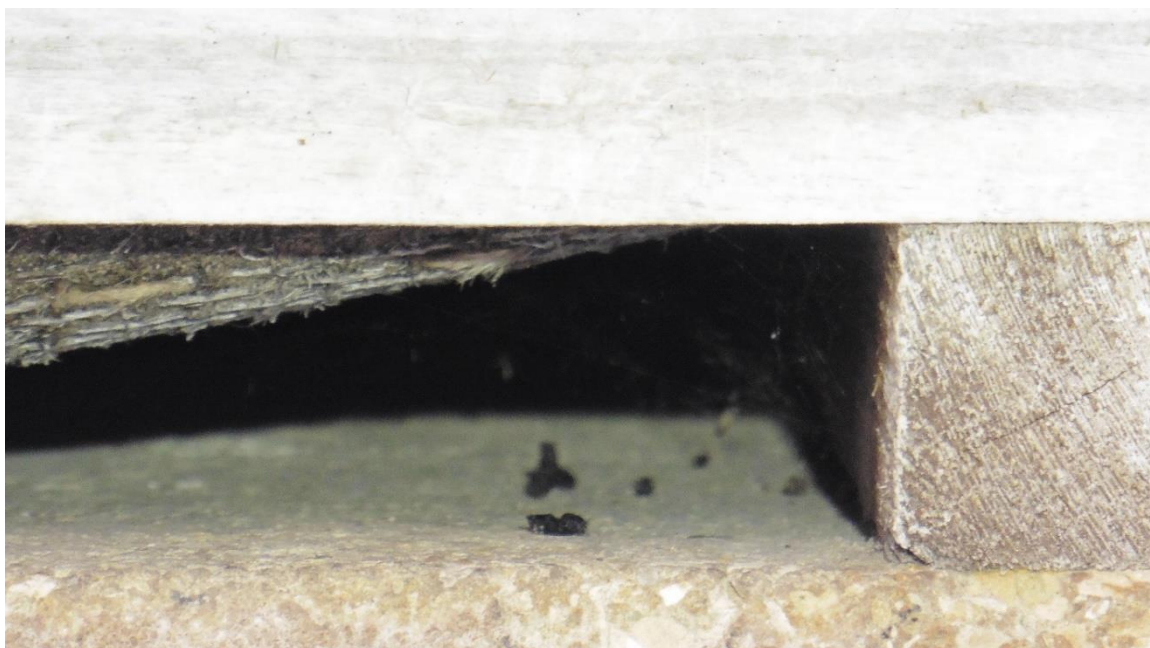
Photograph 6: Dropping evidence from within the void between stone and roofing frame and membrane.
