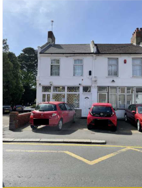
Photograph 01 - Front of Building
