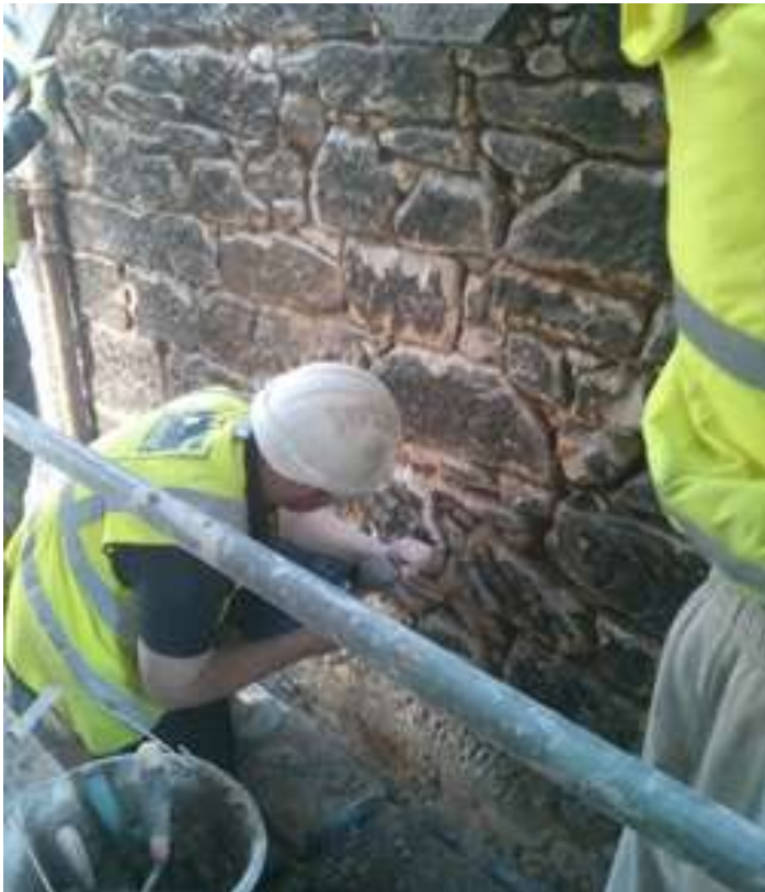
Pointing a rubble wall in a lime-based mortar
