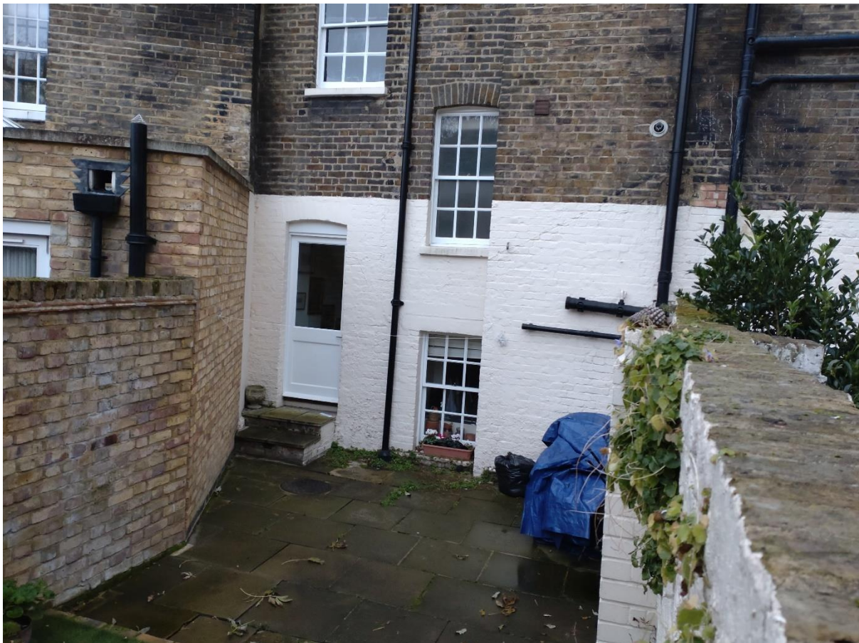
Rear of No. 9
