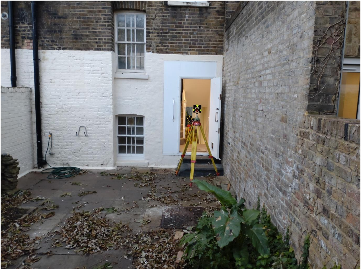
Rear Elevation to No. 9
