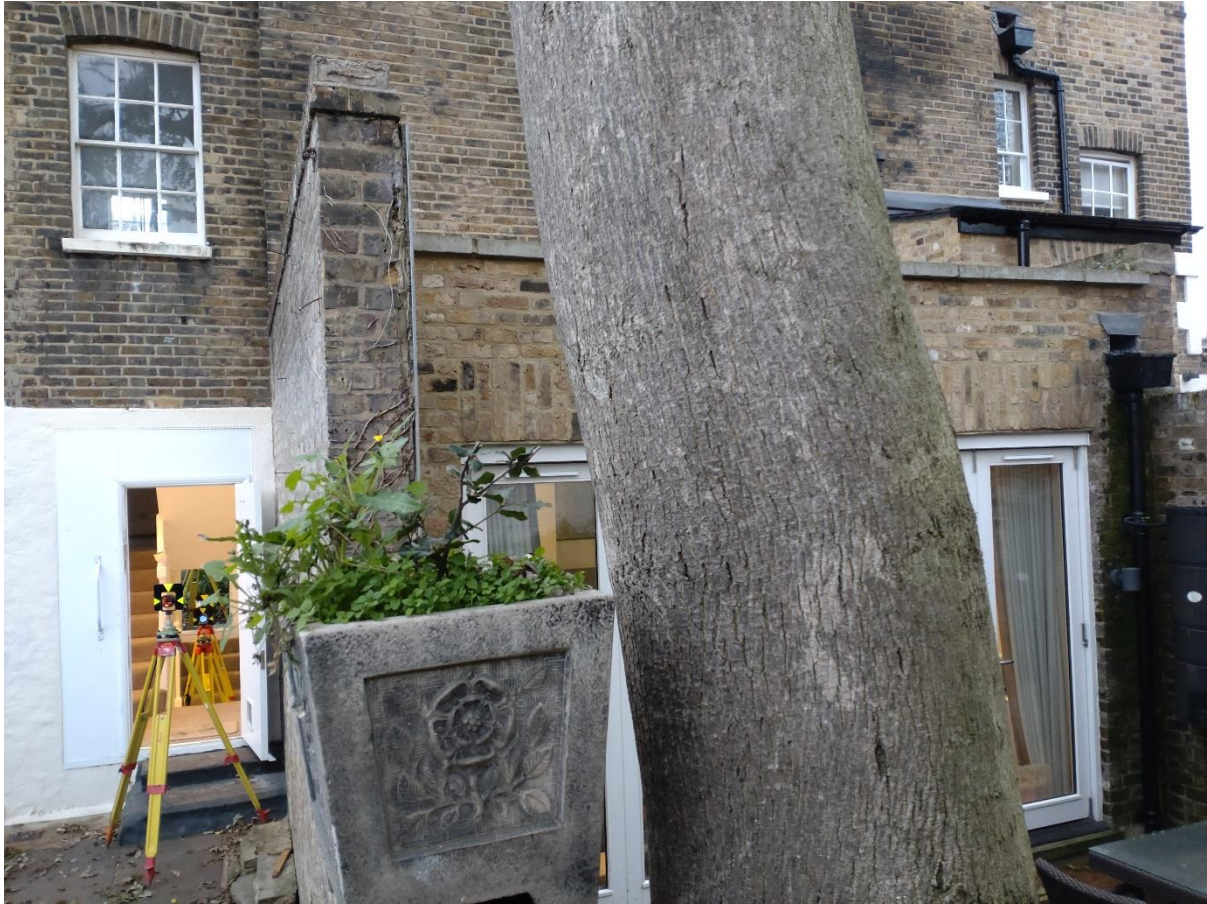
Extension to the rear of No. 7 (completed in 2013)
