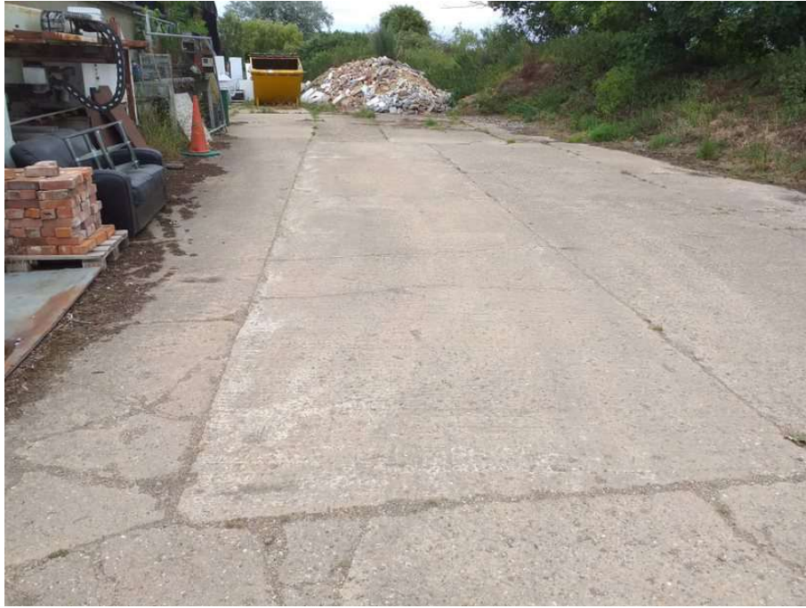
Hard standing slab and mound on eastern boundary
