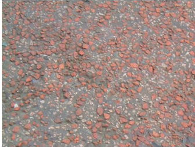
Figure 5 – HRA with red coated chippings
