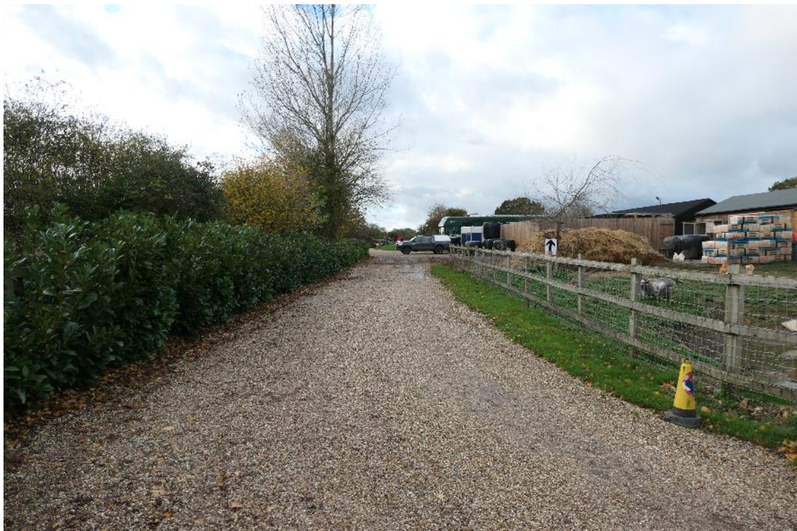
Photo 2 , hardstanding and sp.-poor intact hedgerow along access track, looking west.
