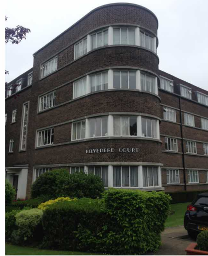
Image 1: Front view of Belvedere Court; Flat 5 is on second floor
