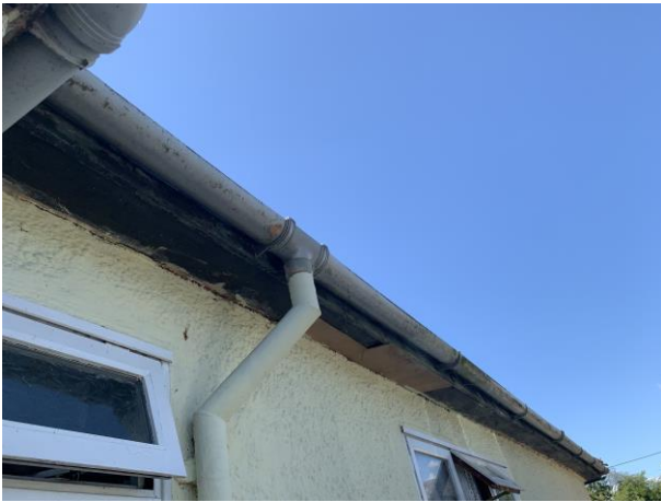
Photo 7: Building 1, soffit box, north elevation.
