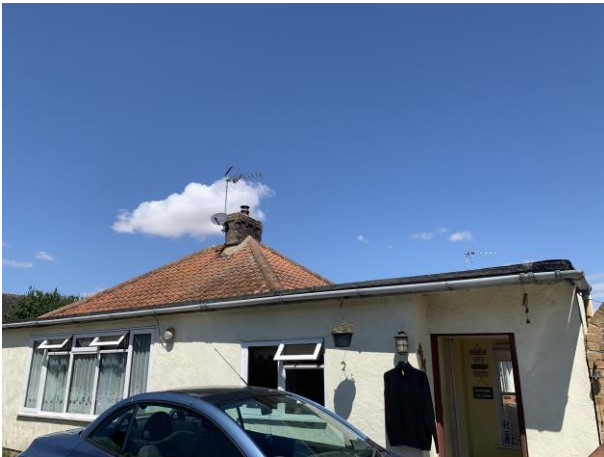
Photo 3: Building 1, south elevation.
