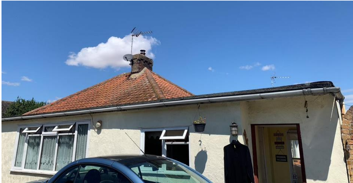
Building 1, Occupied Bungalow Dwelling Onsite.
