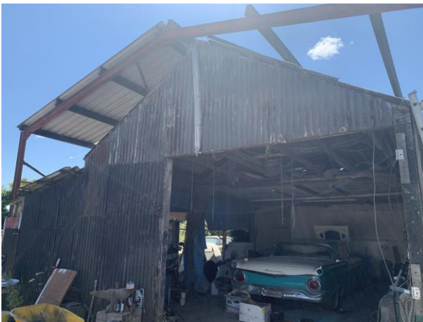
Photo 11: Building 2, north elevation.
