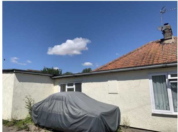
Photo 4: Building 1, south elevation.
