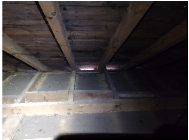
Photo 10: Building 1, loft void. Light ingress.
