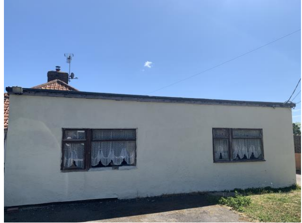
Photo 2: Building 1, west elevation.
