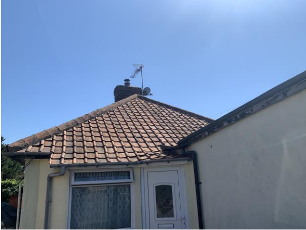
Photo 1: Building 1, west elevation.
