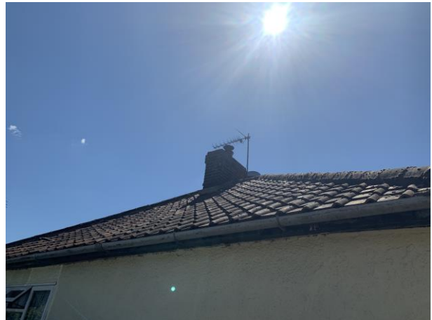
Photo 6: Building 1, north elevation.
