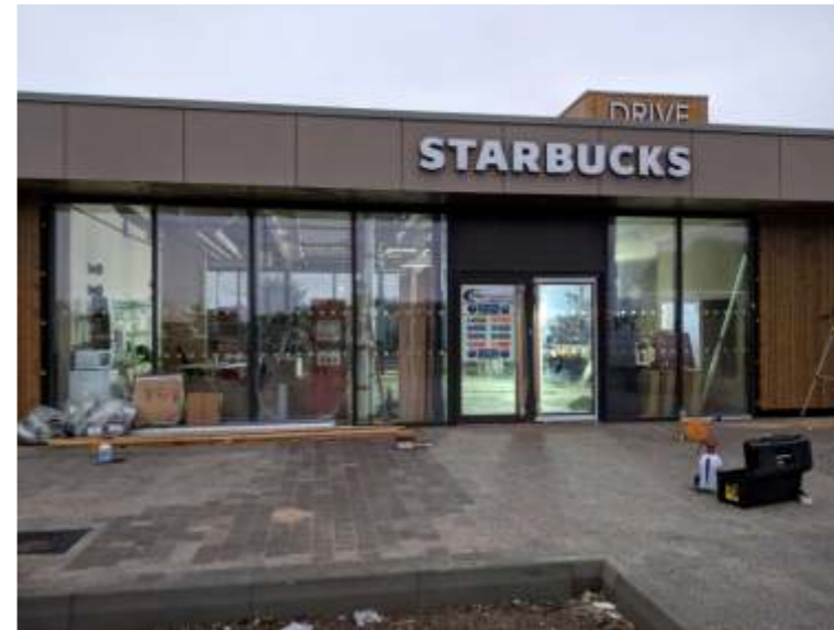
Photo example of sign
