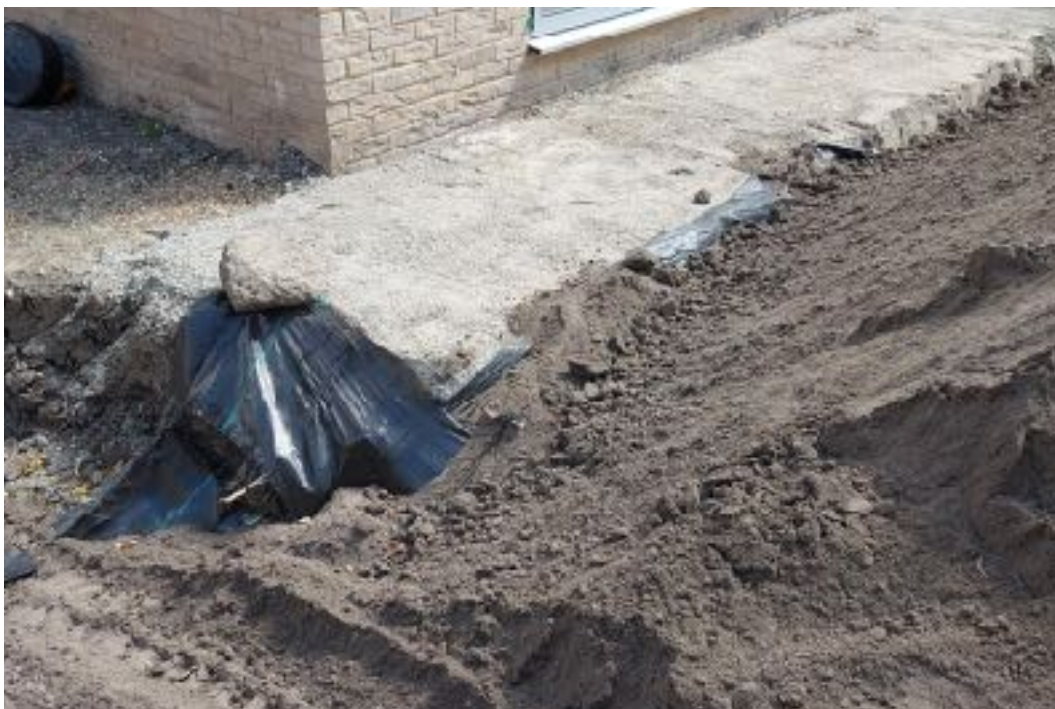
100mm concrete/ 600mm topsoil
