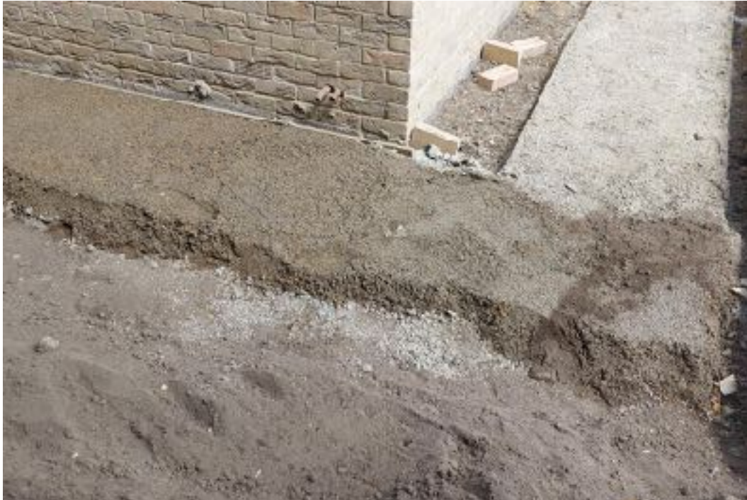
100mm concrete/600mm topsoil
