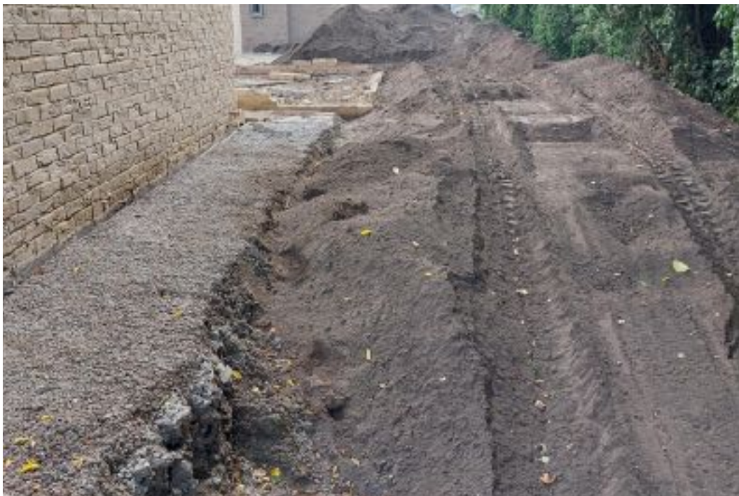
100mm concrete/600mm topsoil
