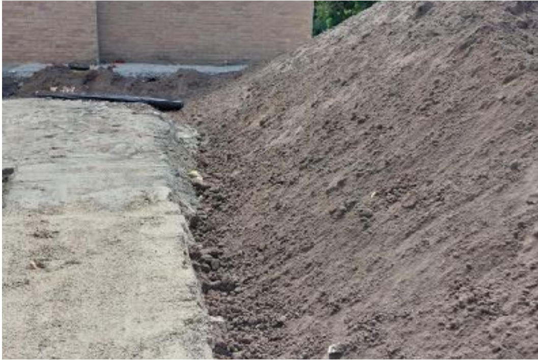
100mm concrete capping/ 600mm topsoil
