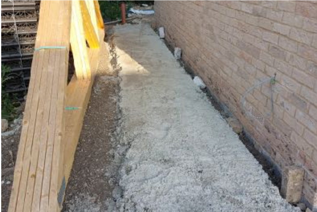
100mm concrete capping under hard landscaping
