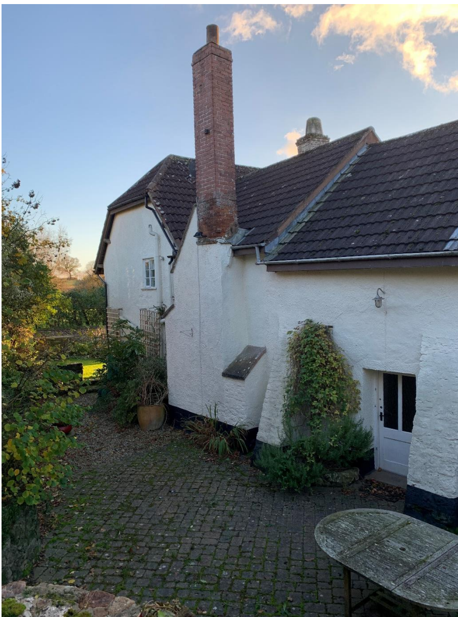
Figure 1: chimney to be reduced in height
