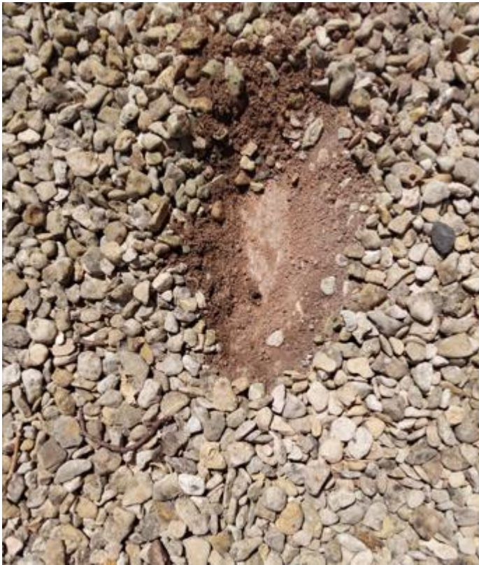
Photograph 5: Hardstanding beneath gravel surfacing across the area
