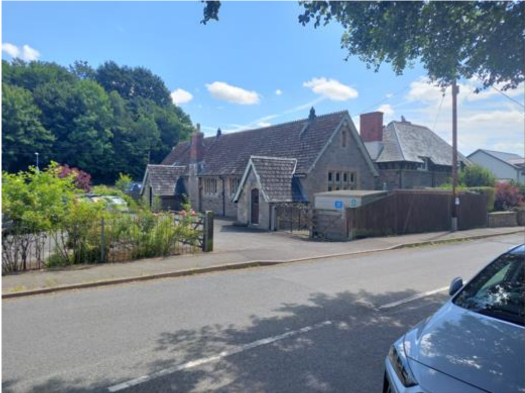
Photograph 1: General view of site
