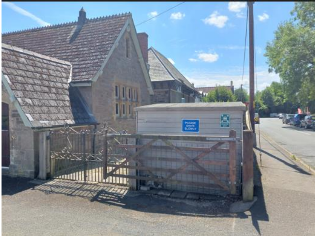
Photograph 2: View of access gates to patio area
