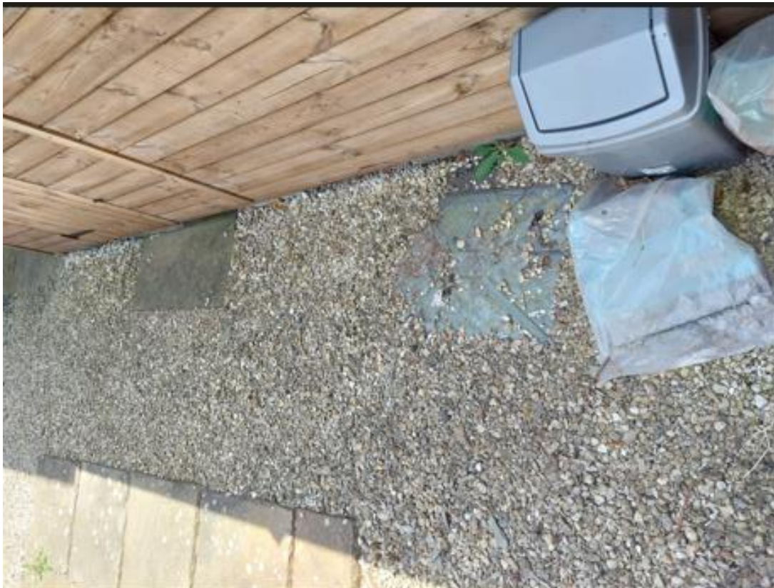
Photograph 6: Drain cover in front of remaining shed
