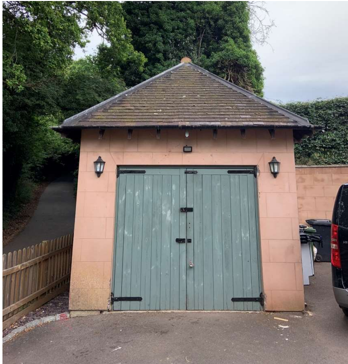
Existing South elevation of garage.
