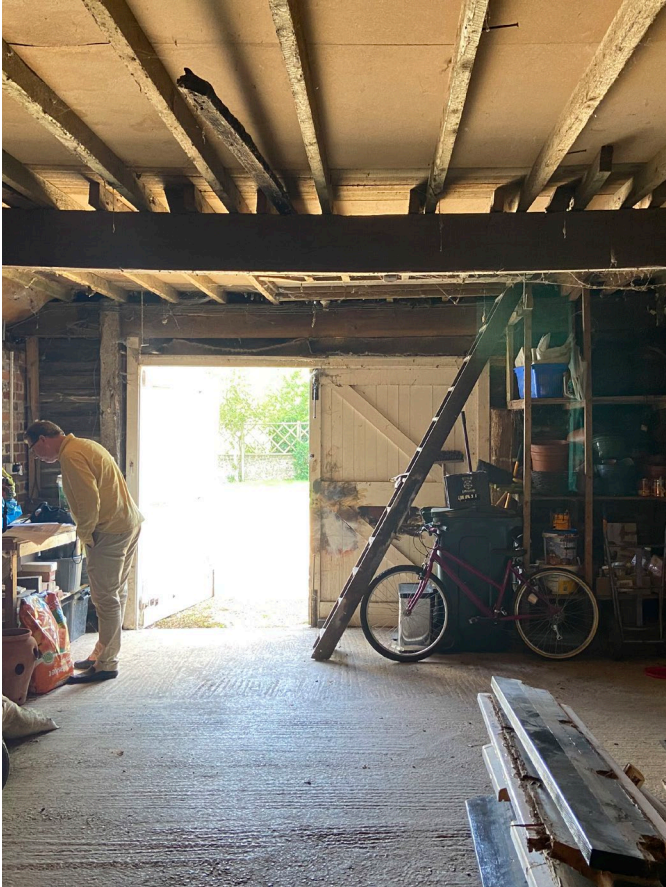
Figure 15: Barn East Elevation Internal
