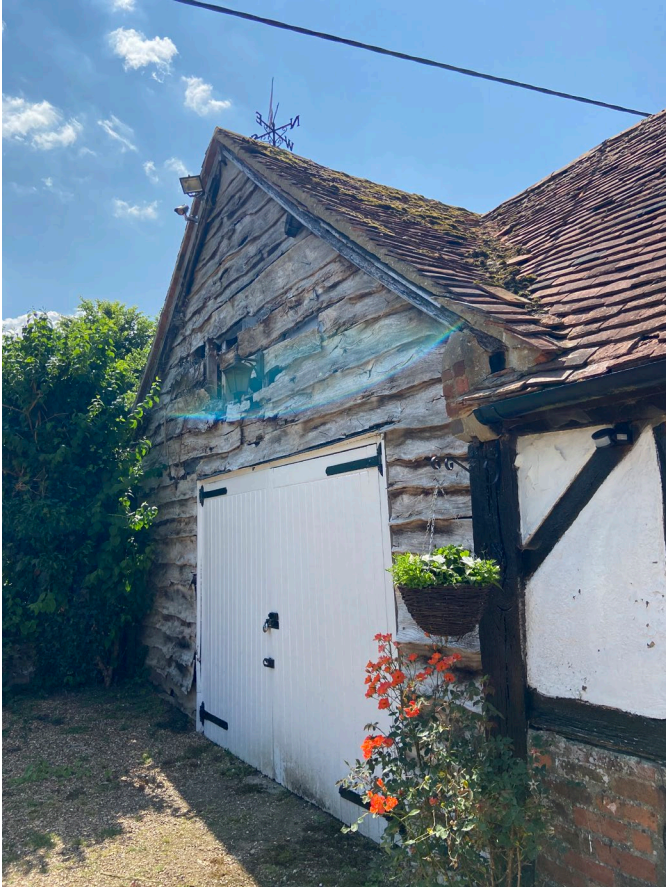
Figure 12: Barn East Elevation
