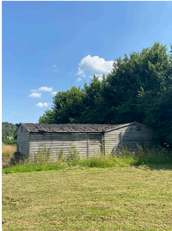
Figure 19: Stables West Elevation
