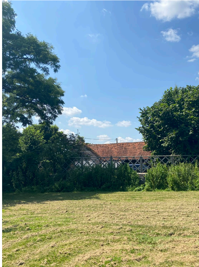
Figure 22: Brick Wall Access (Stables Side)
