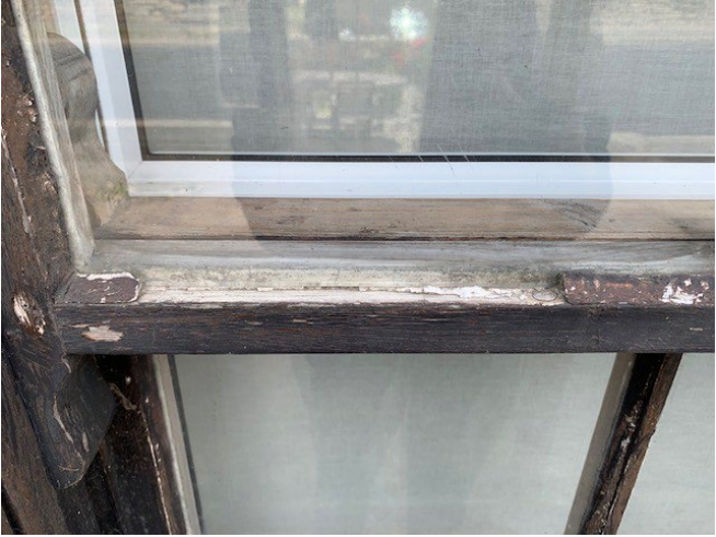
The bottom windows all have loose & putty missing. Paintwork on all windows in a bad state
