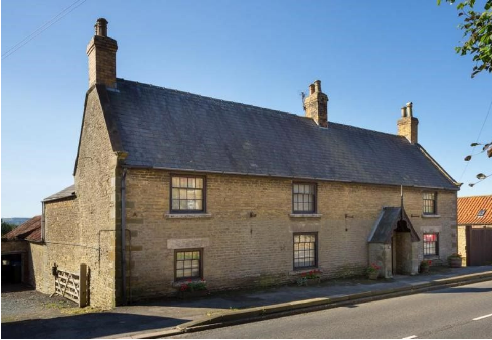
The front of the house – all window lintels and woodwork to be painted
