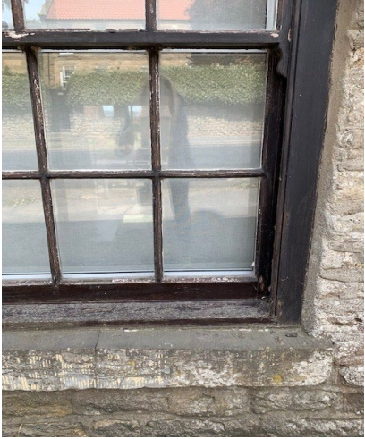
The bottom windows all have loose & putty missing. Paintwork on all windows in a bad state
