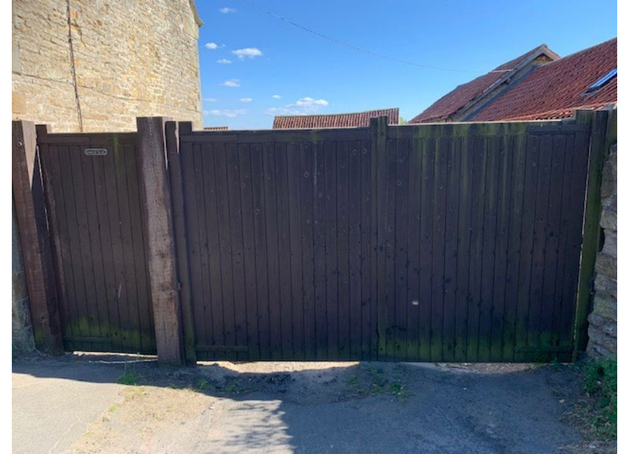
The main gates – all woodwork to be painted
