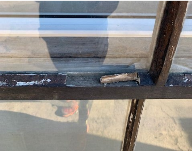
The bottom windows all have loose & putty missing. Paintwork on all windows in a bad state
