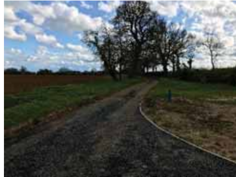
Photo 8: View south along Leys Lane, site access road.
