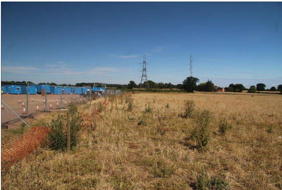
Plate 4: View of construction within the southwest of the site, looking northwest
