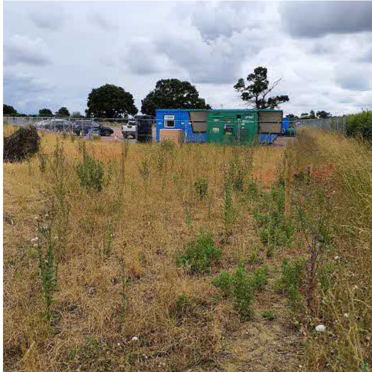
Photo 5. View from the north of construction compound in SW corner of redline area.
