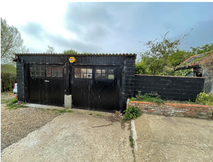
Figure 3 – Double garage to be demolished
