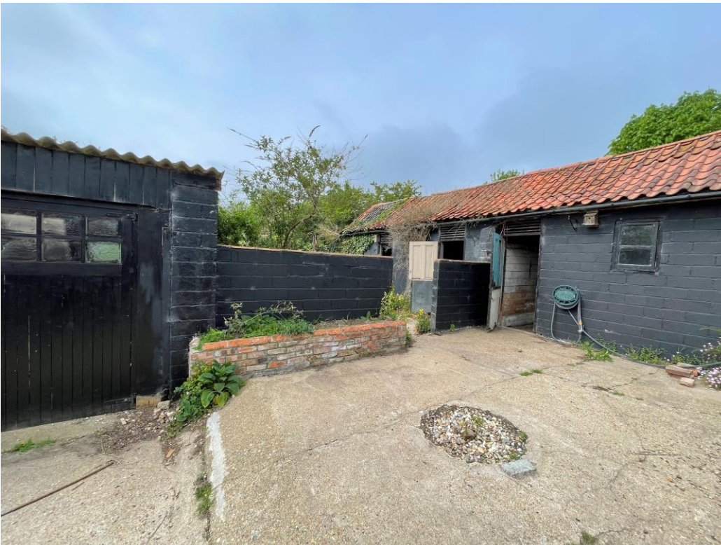
View looking towards courtyard area (west)
