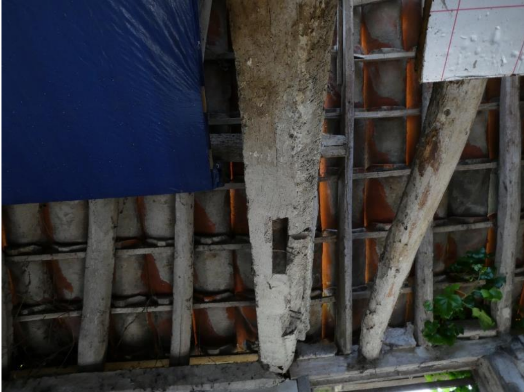
Photo 13 , example mortis and tenon joint which are exposed to high levels of natural daylight.
