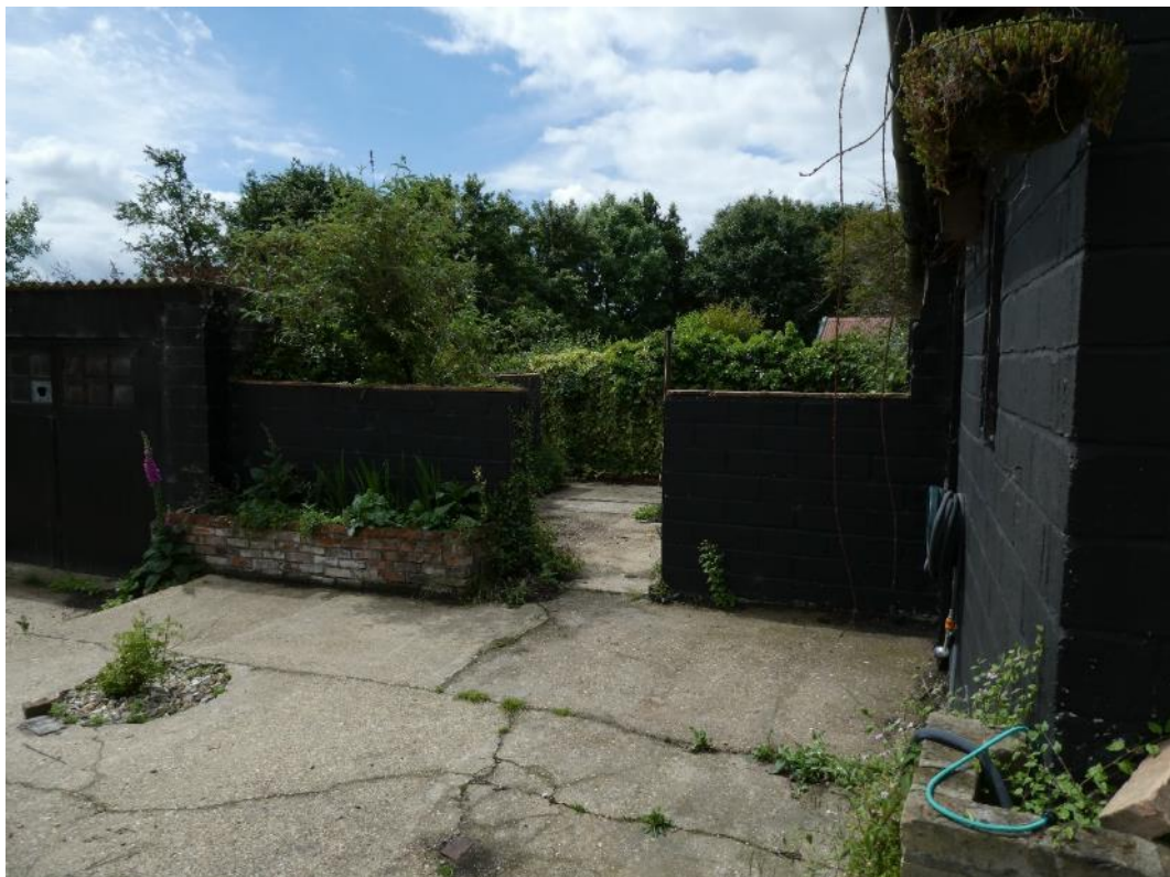
Photo 2 , hardstanding and brick wall between outbuildings, looking southwest.
