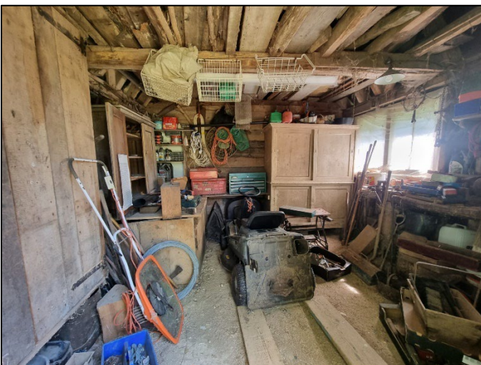
c) Ground floor interior
