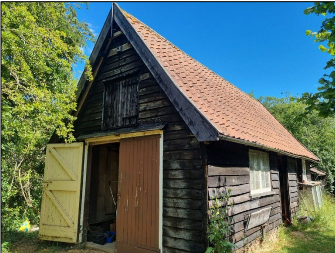
b) Southern/western aspect of the barn
