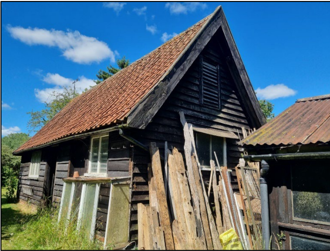
a) Eastern/southern aspect of the barn
