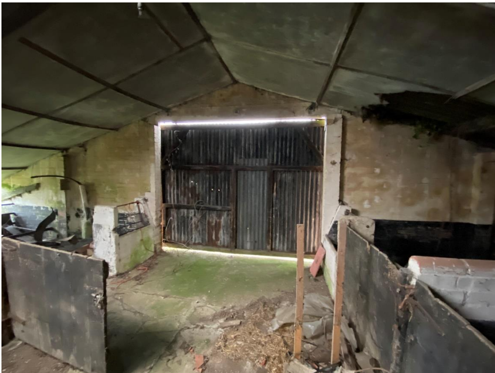
8. Rear internal view
