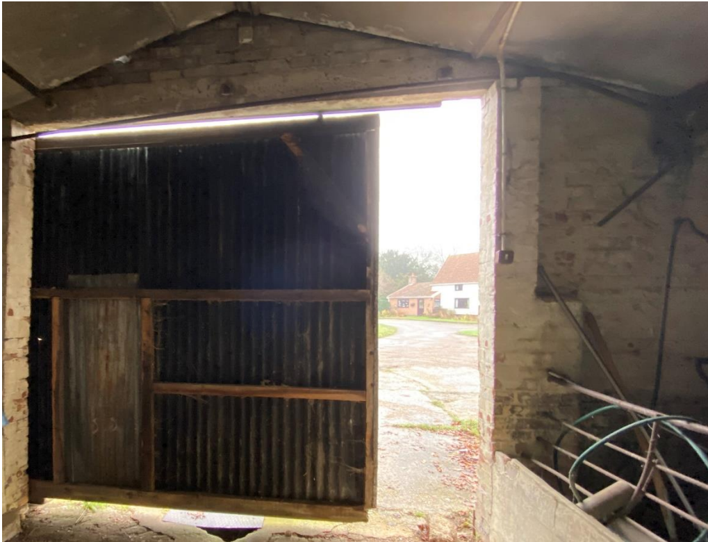
5. Front internal view
