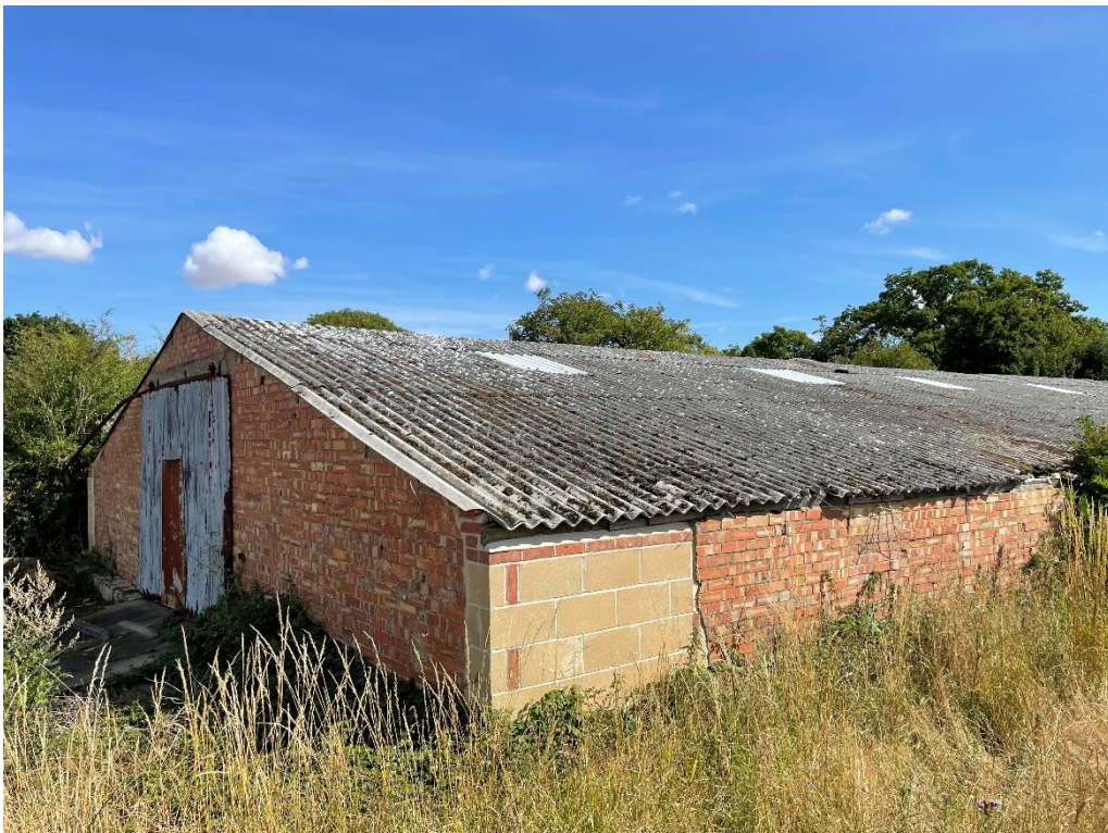
4. Left hand external view from rear corner
