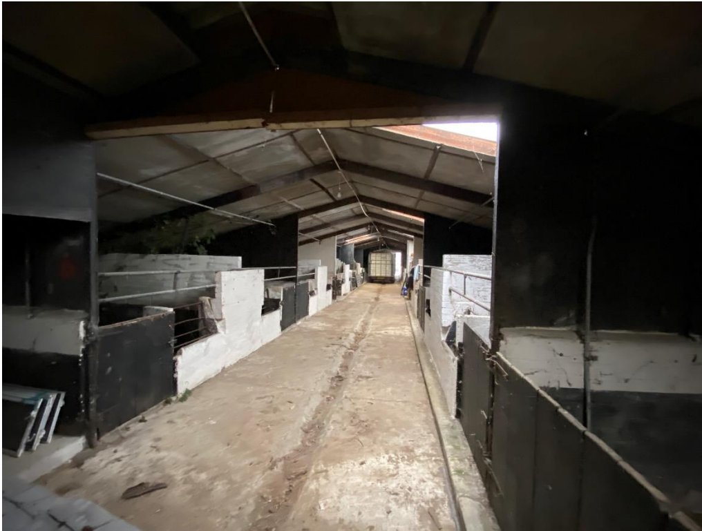
7. Internal view looking towards front
