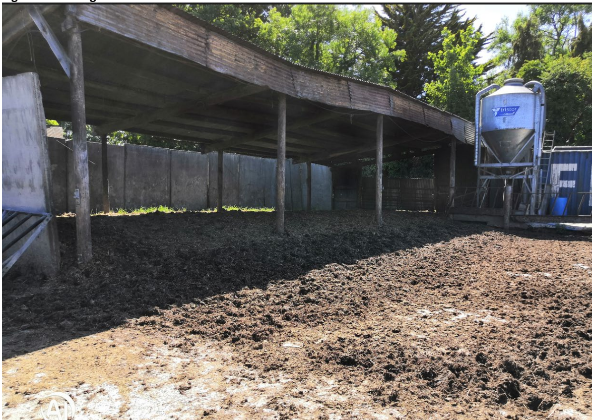
Figure 4: Existing cattle shed to west
