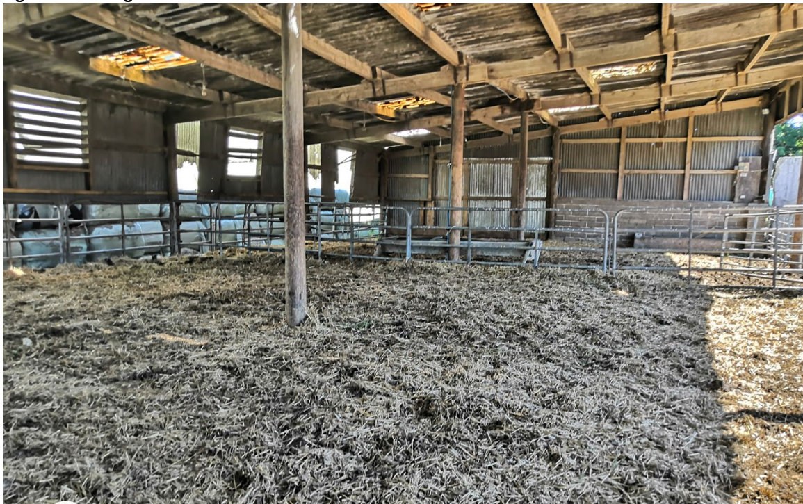
Figure 5: Existing cattle shed to east
