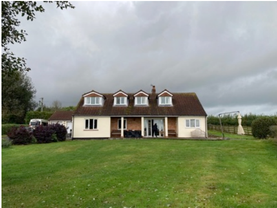
House from garden – East façade – untidy roofscape
