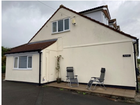
South façade – unwelcoming at present
