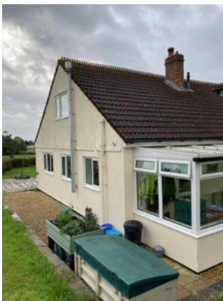
House from the North West showing conservatory and aga flue to be removed
