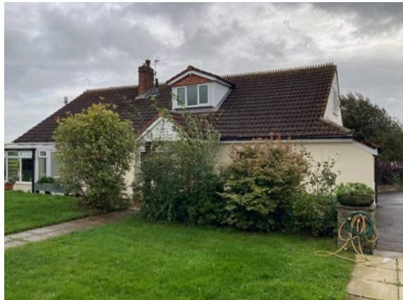
West façade – 'front' entrance difficult to find.
