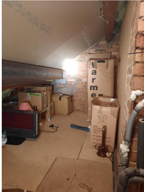
Plate 6: Side loft against chimney breast.
