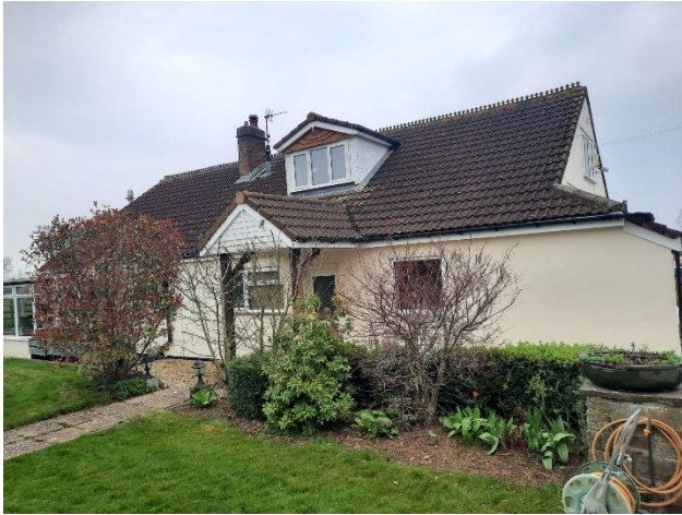
Plate 1: Northwest elevation and garden.
