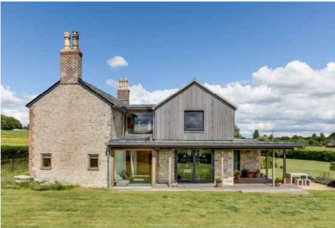
Image reference - 1st floor vertical timber cladding
