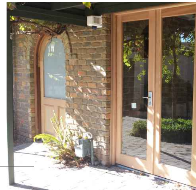
Timber french doors and windows
