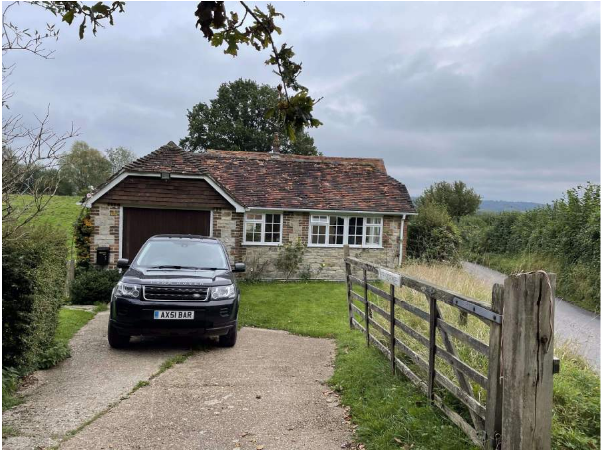
West elevation of garage building
