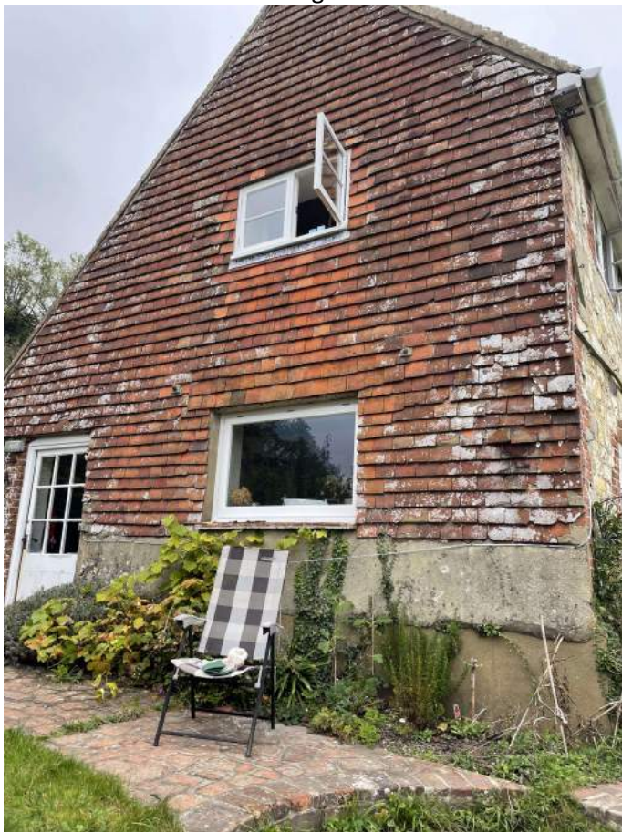
South elevation of the dwelling
