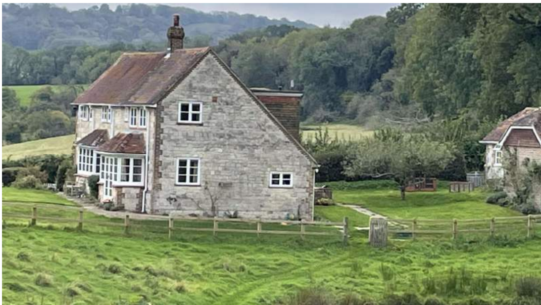
North elevation of the dwelling
