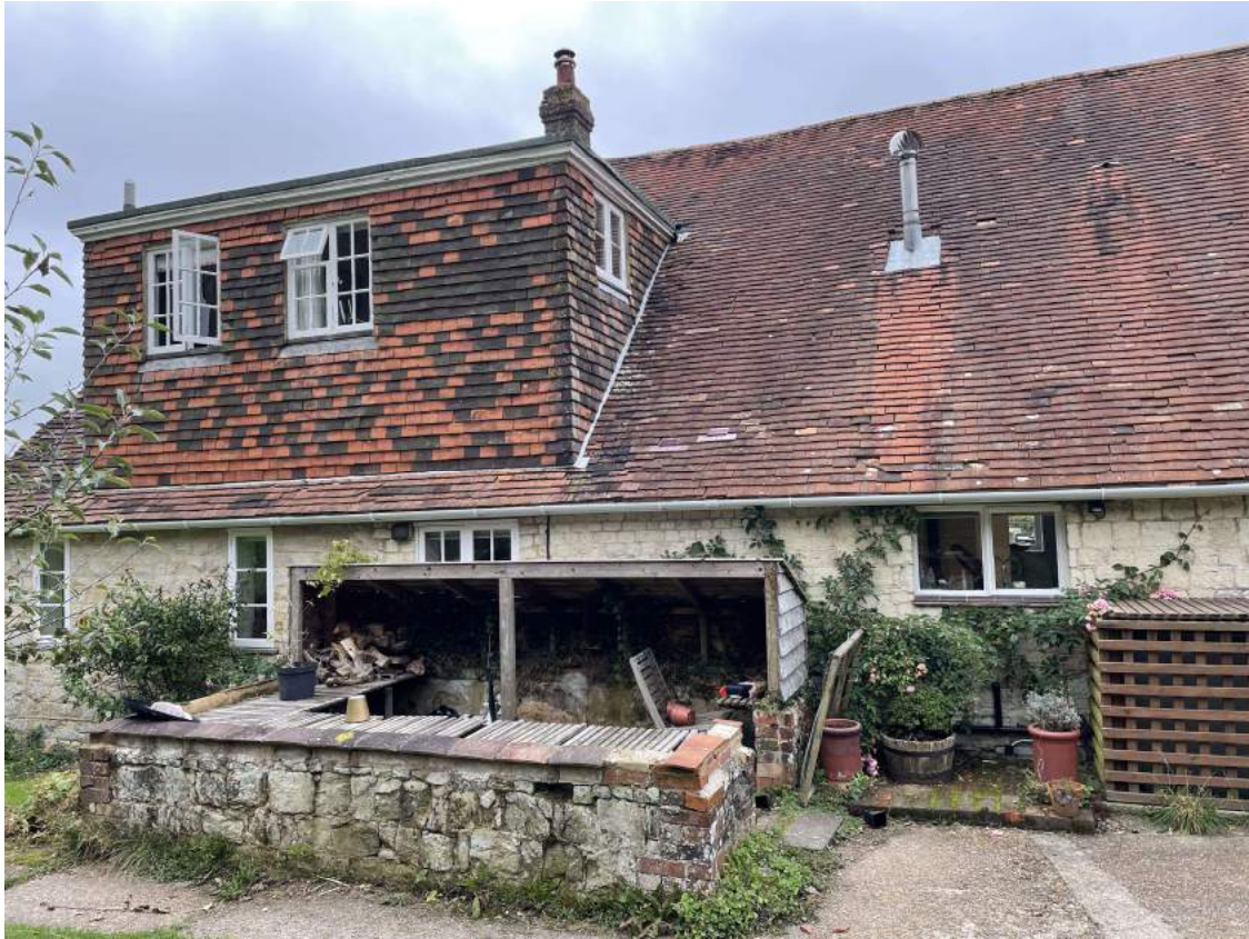
West elevation of the dwelling
