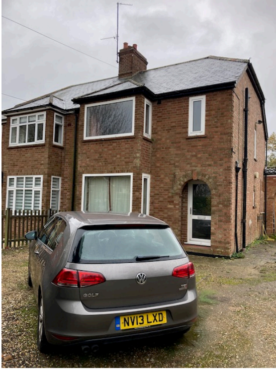
Top left: view to the front of the house
