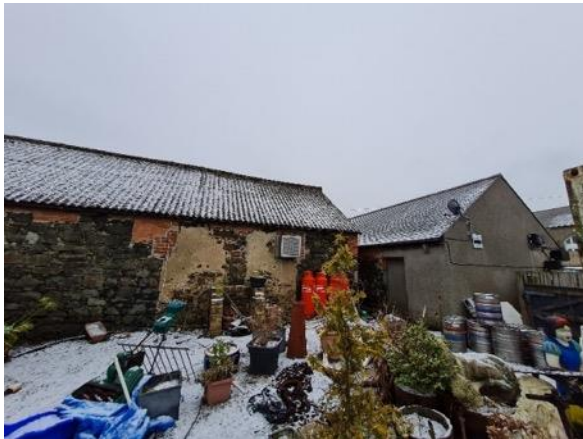
Figure 9: Outbuildings - north/rear elevation.
