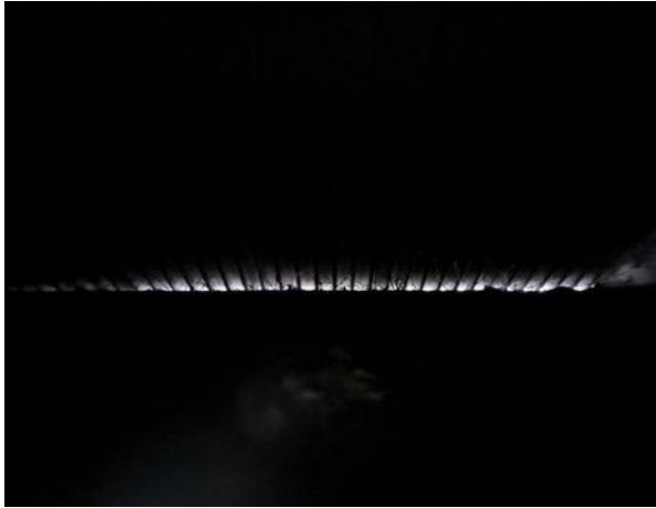
Figure 21: Outbuilding - loft - light entering underneath the end of corrugated asbestos roof.
