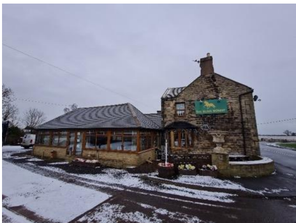
Figure 13: B1 - conservatory - west elevation
