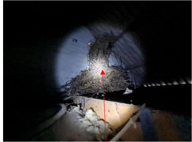
Figure 22: Outbuilding - loft - jackdaw nest.
