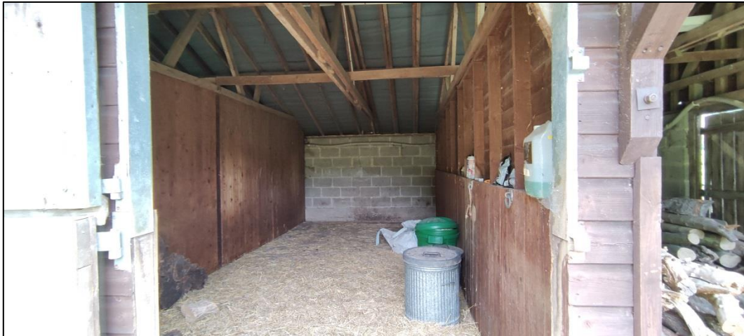
Figure 49 – Showing timber walls partitioning the interior of the stables
