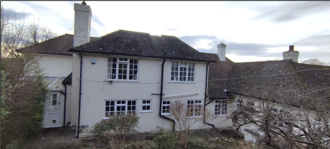
Figure 4 – Side (north-eastern) elevation of Orchard Cottage showing single storey extensions
