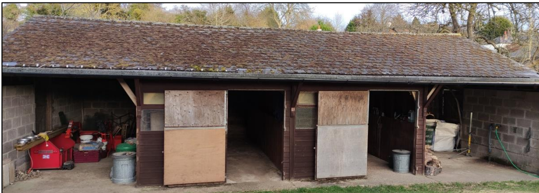
Figure 51 – showing open sided nature of the stable block and slate roof
