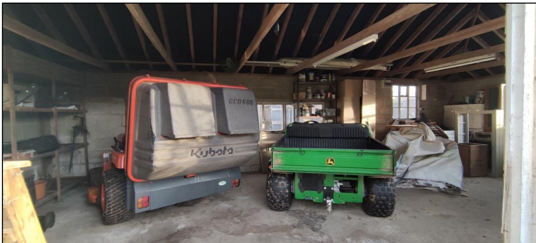
Figure 32 – showing large internal void, with no separate roof void and farm equipment
