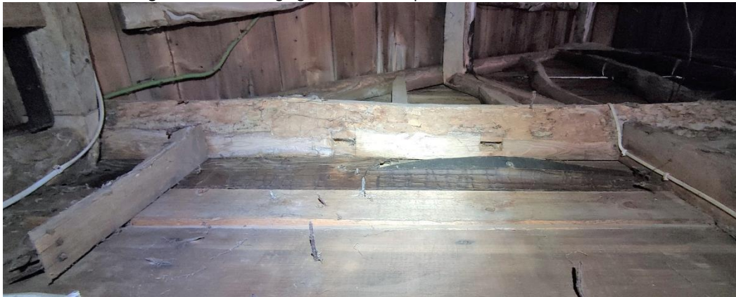
Figure 40 – showing notches in the hand-hewn timbers that could be utilised by bats
