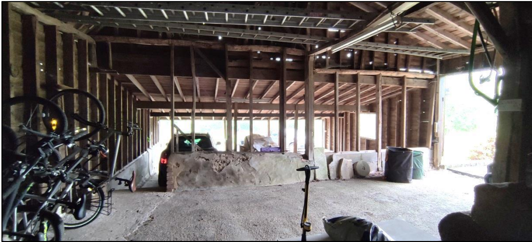
Figure 39 – showing light levels and open sides around the barn
