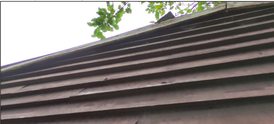
Figure 53 – showing tightly fitting weatherboarding found on majority of the building
