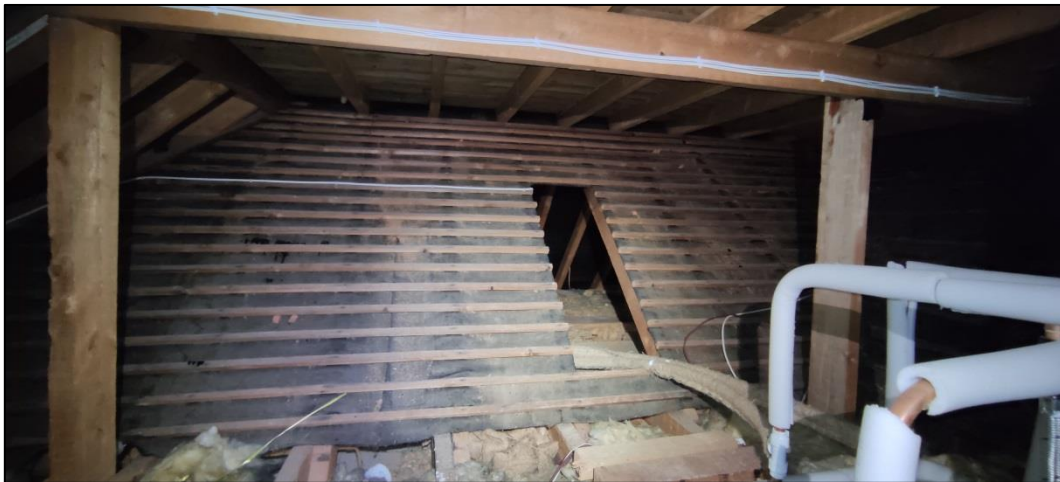
Figure 15 – showing roof void 1, with previous section of roof and boarded section
