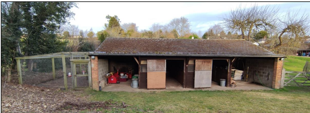
Figure 12 – south-western elevation of the stables, open to the environment
