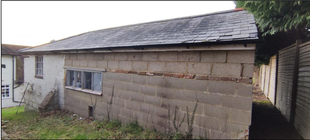
Figure 35– showing breeze-block construction and proximity to fence and trees
