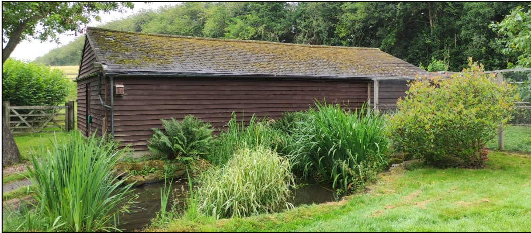
Figure 13 – rear (north-eastern elevation) of the stables with weatherboarding
