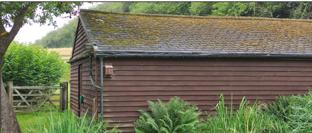
Figure 52 – showing slate tiles and weatherboarding covering the external walls
