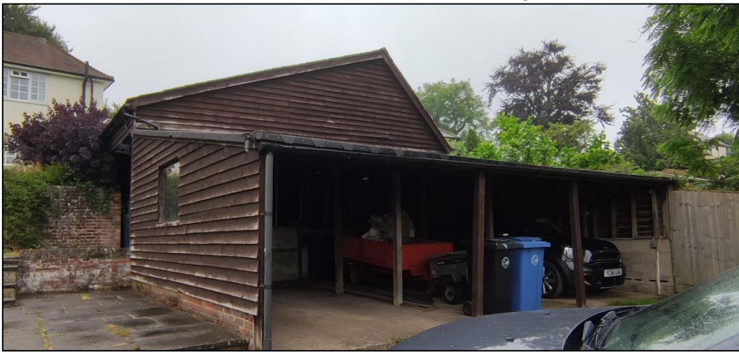
Figure 11 – newer section (south-western elevation) of the Garage/Barn with bitumen felt roof
