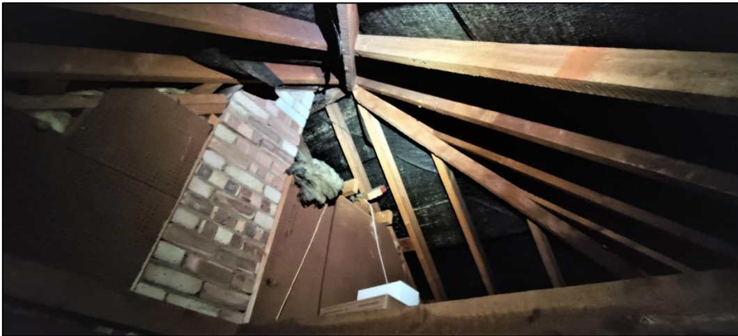
Figure 18 – showing hipped section, chimney and bitumen underlay
