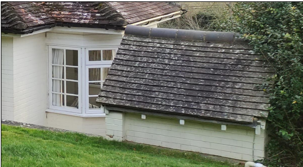
Figure 7 – Side (north-western) elevation of the Coal Shed
