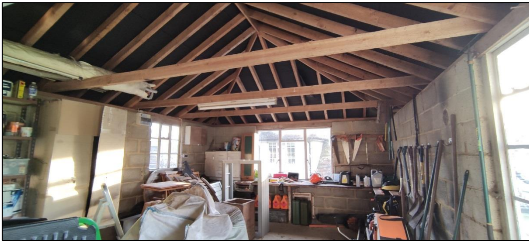
Figure 33 – showing internal light levels, modern timber trusses and single glazed windows
