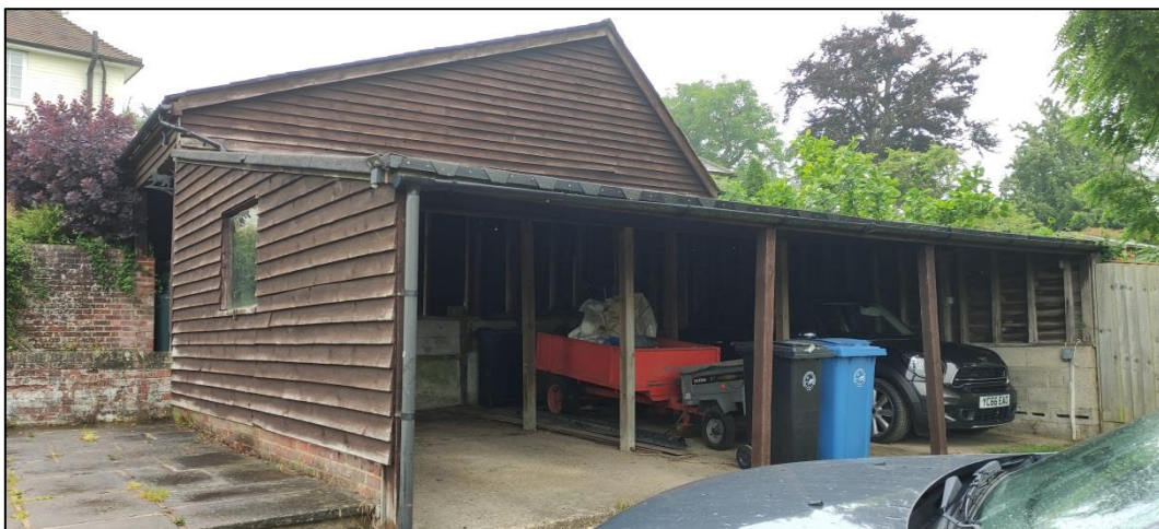
Figure 45 – showing open end used as a garage and weatherboarding on the exterior
