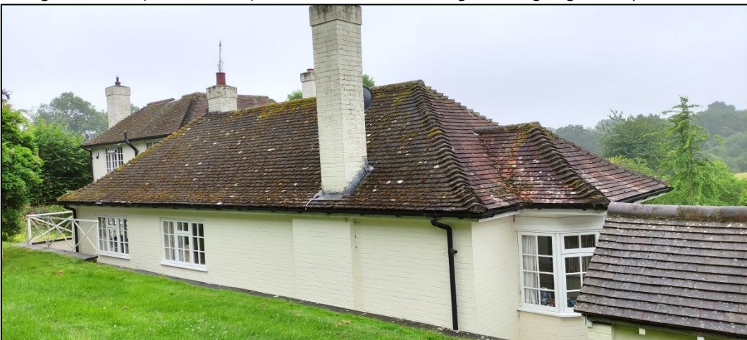
Figure 5 – Side (north-western) elevation of Orchard Cottage showing external chimney
