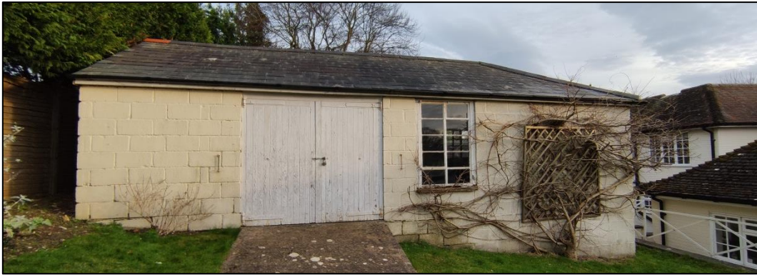
Figure 8 – Front (north-western) elevation of the Tractor Shed
