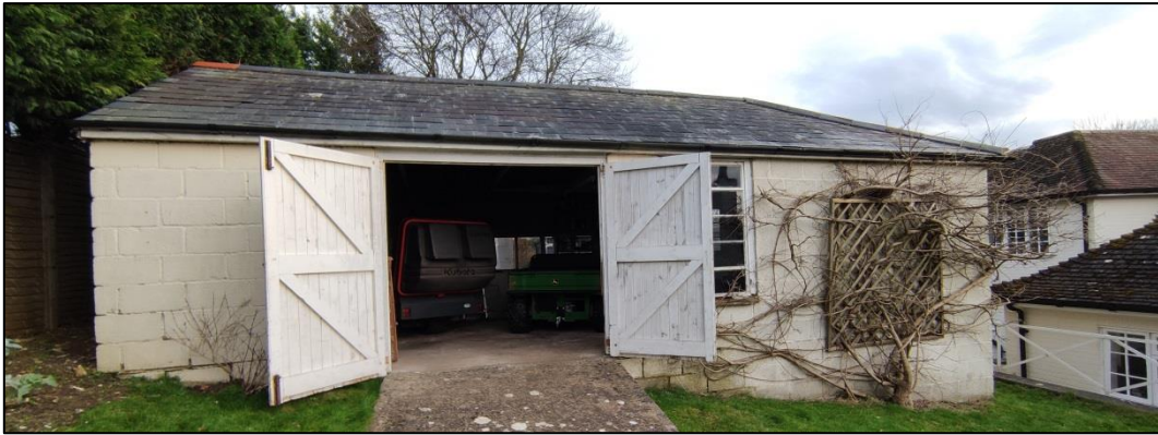
Figure 34 – showing large double doors, slate roof and single glazed windows
