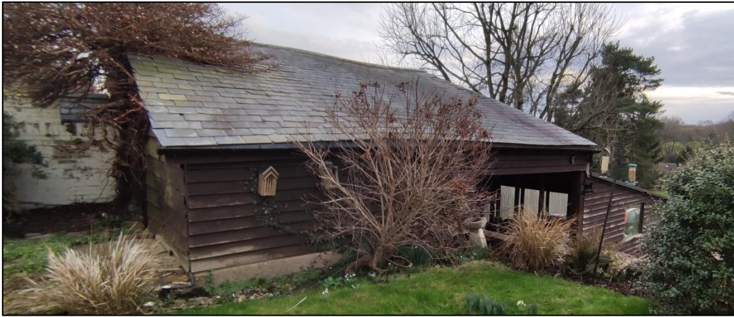
Figure 10 – older section (north-western elevation) of the Garage/Barn with slate tiled roof
