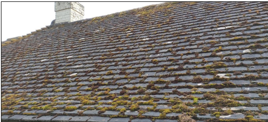
Figure 27 – roof showing machine-made, concrete tiles, chimney and hip bonnet tiles
