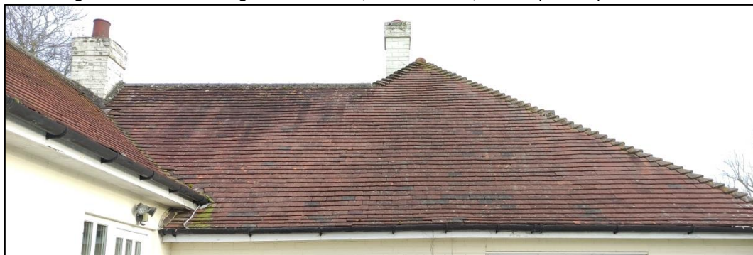
Figure 28 – image showing machine-made clay tiles, hopped sections, valleys and chimneys
