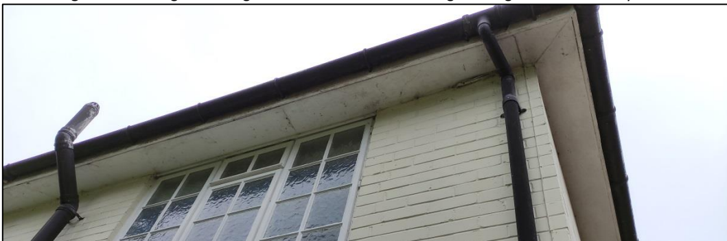
Figure 31 – showing sealed eaves around the building
