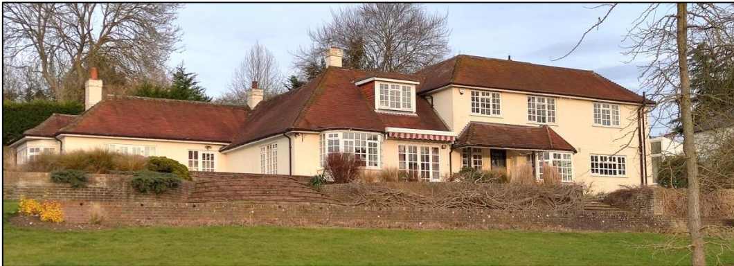
Figure 3 – Rear (south-western) elevation of Orchard Cottage showing single storey extensions
