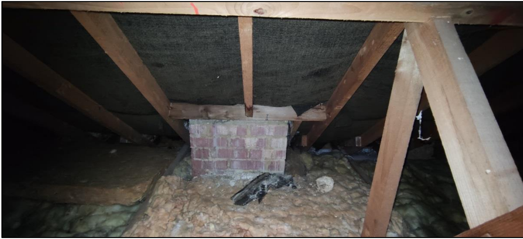
Figure 23 – chimney stack in the western-most section of the roof void
