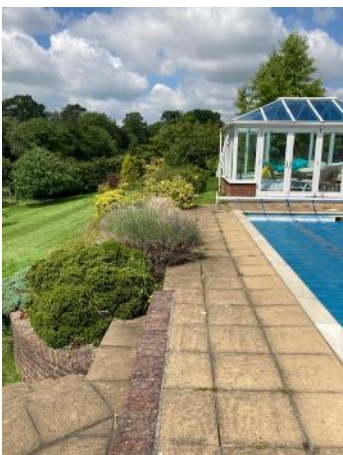
Figure 5. Hardstanding paving around swimming pool.
