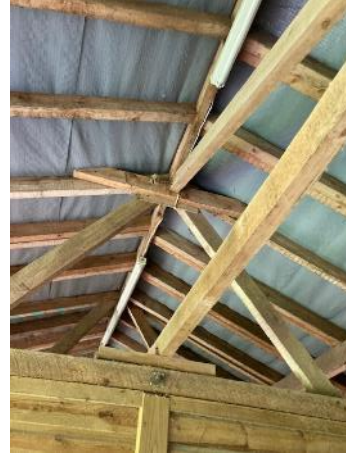
Figure 55. Interior of B6 showing plastic roof underlay and beam structure.
