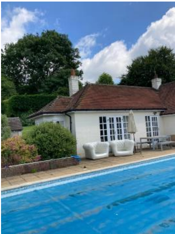
Figure 20. B1, north eastern corner.
