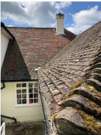
Figure 22. B1, north eastern aspect, central area.
