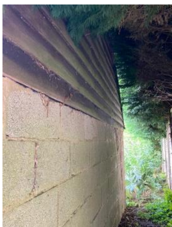
Figure 40. B4, northern aspect. Note wooden cladding with gap at base.
