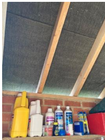
Figure 37. B3, interior showing open eaves.
