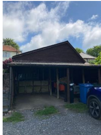
Figure 45. South western aspect of B5.
