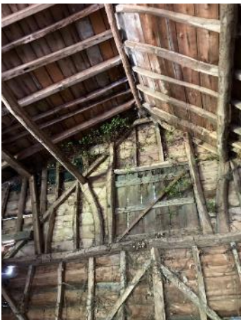
Figure 50. Interior of B5 showing north eastern gable wall.
