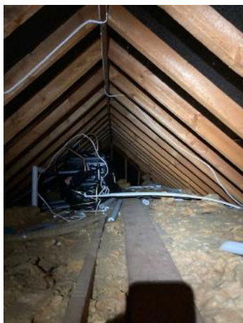
Figure 32. Loft void 2, B1.
