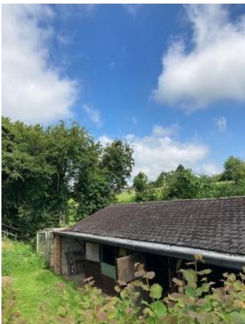
Figure 52. B6, south western aspect.
