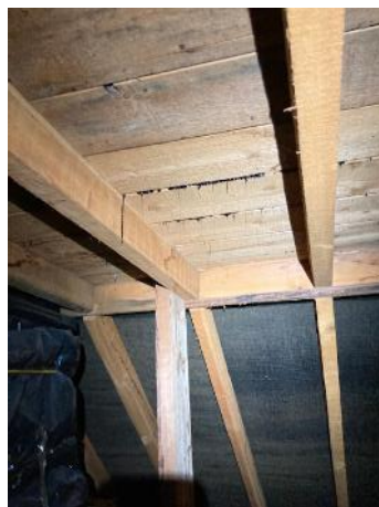
Figure 33. Flat roof section of loft void 2, B1.
