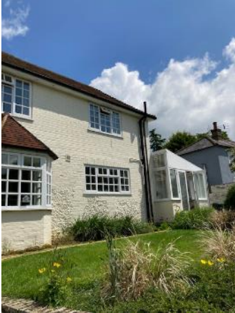
Figure 18. B1, southern end of south western aspect.
