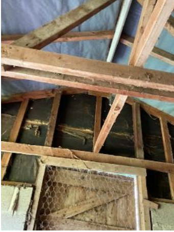
Figure 54. Interior of B6, north western gable end.
