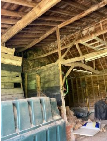
Figure 48. Interior of B5.
