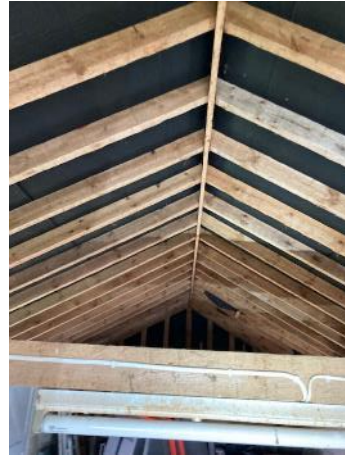
Figure 43. Interior roof structure of B4.
