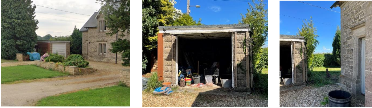
Existing images of the garage to be demolished
