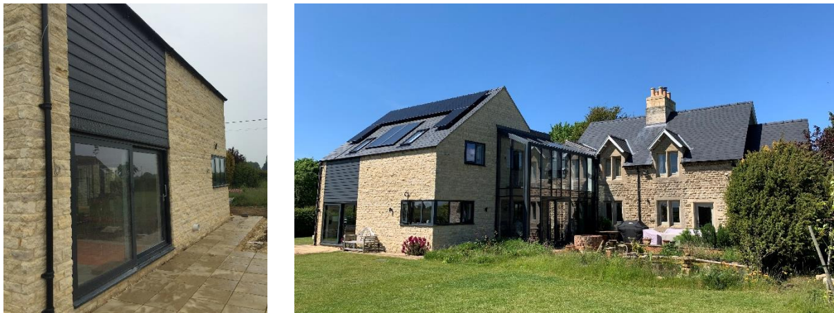
Existing images of the existing extension where the proposed solar canopy will be situated
