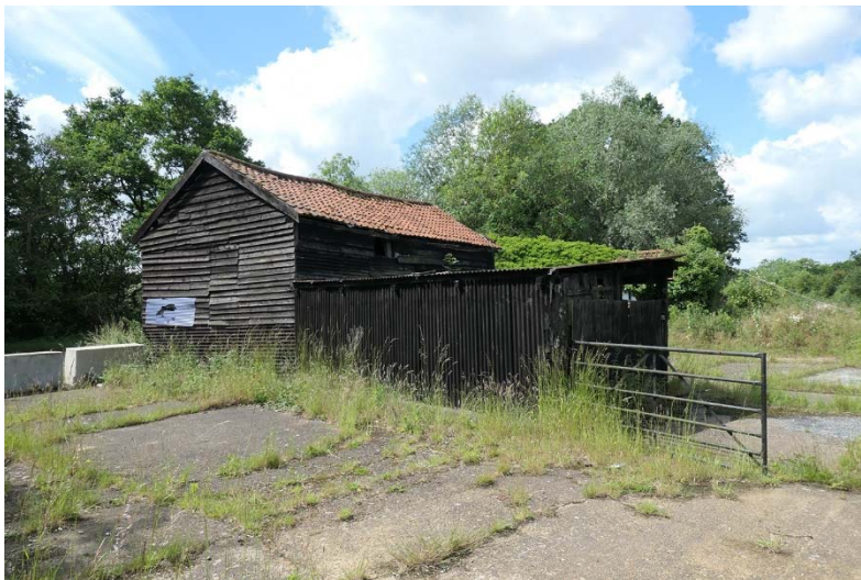
Figure 49 (above). Front (roadside) Elevation. Now blank boarding, the framing above the concrete indicates possibly a blocked midstre opening.
