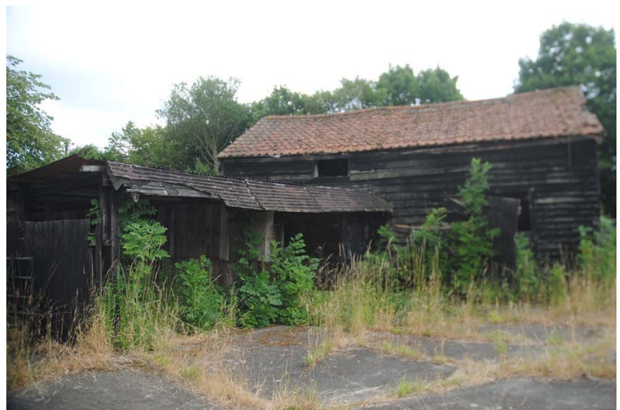
Figure 51 (right). Courtyard elevation of Barn 2 beyond C20 shelter shed
