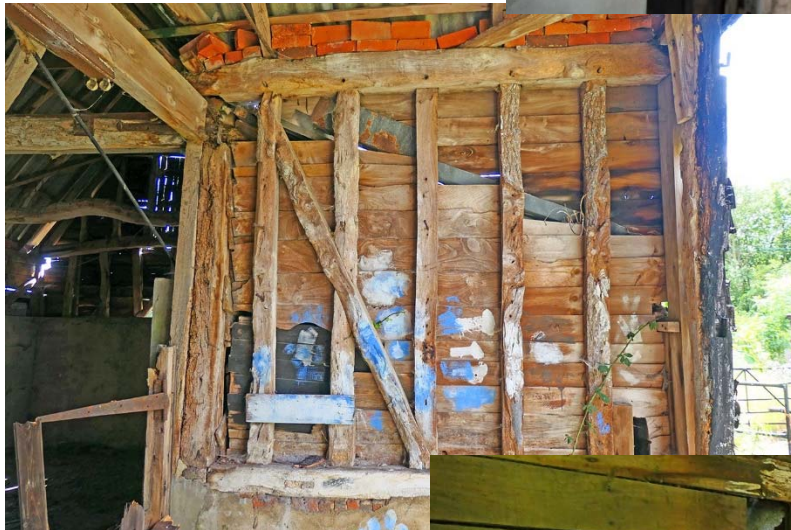
Figure 45 (right). Damage in one of the areas of where there have been longstanding water leaks. High brick plinth using C17 bricks. The C20 blockwork internal casing can be seen beyond.
