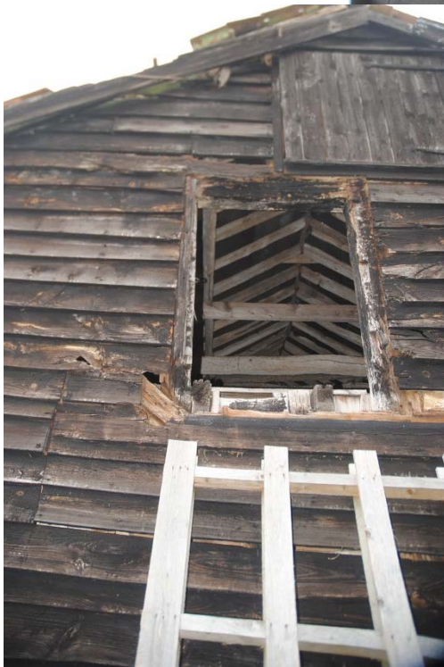
Figure 54 (left). First Floor hatch in West Gable, showing roof structure.
