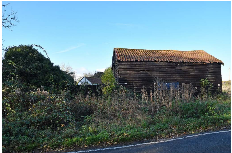
Figure 49 (above). Front (roadside) Elevation. Now blank boarding, the framing above the concrete indicates possibly a blocked midstre opening.
