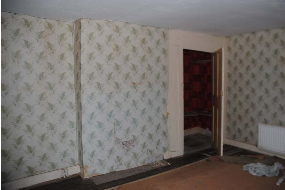
Figure 30. Bedroom 1 with typical simple details and blocked fireplace. C18 cupboard.
