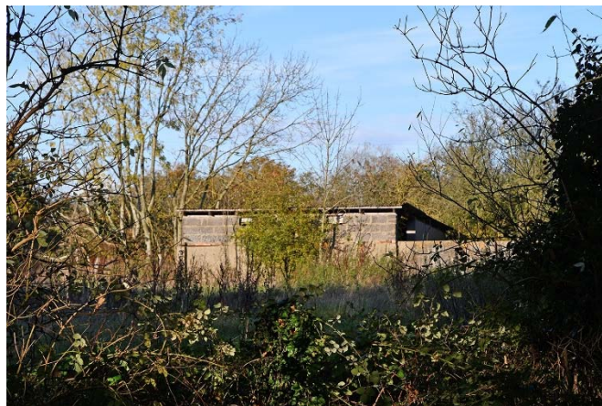
Figure 62. View across the Western field from Chelmsford Road, showing these mid-C20 blockwork units.
