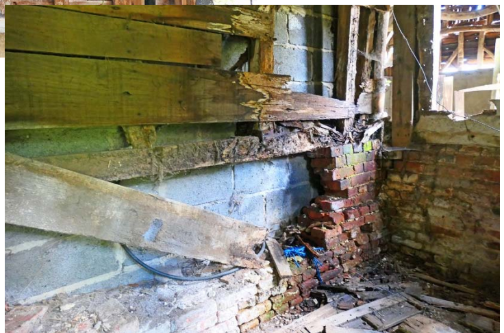
Figure 45 (right). Damage in one of the areas of where there have been longstanding water leaks. High brick plinth using C17 bricks. The C20 blockwork internal casing can be seen beyond.
