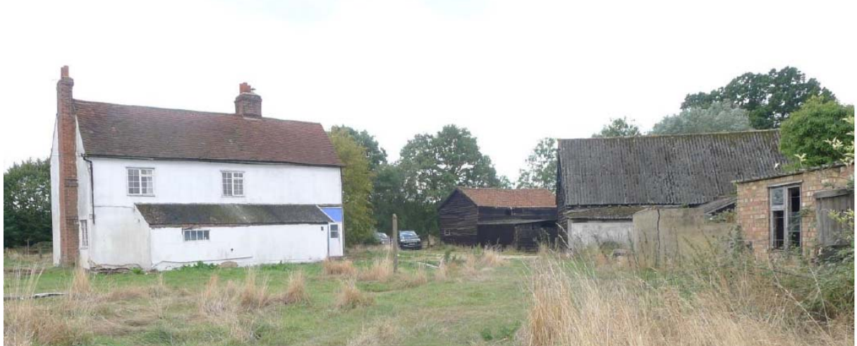
Figure 23. Rear and East Elevations of Farmhouse, with Rear of farmbuildings beyond (2016).
