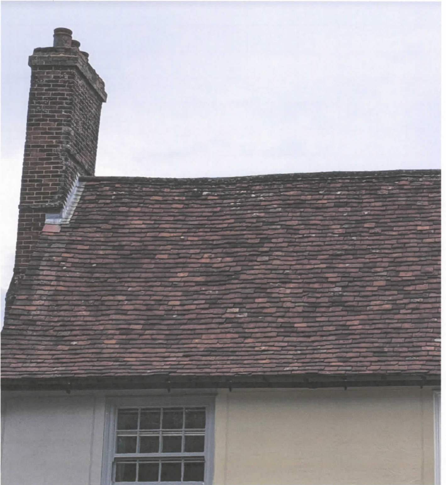
Suggested replacement tile as suggested by the roofer.
