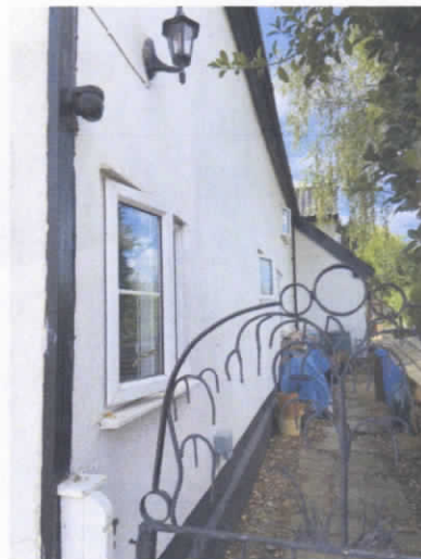
Photo 31: N elevation, bitumened 16C brick plinth
