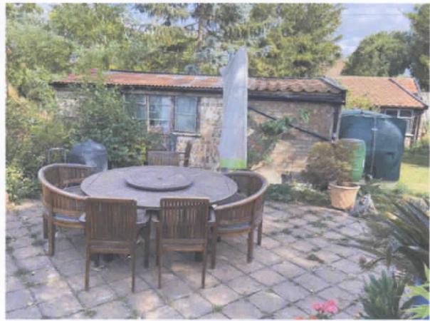
Photo 15: shed, W side, roof pantiled on S part and corrugated on N part
