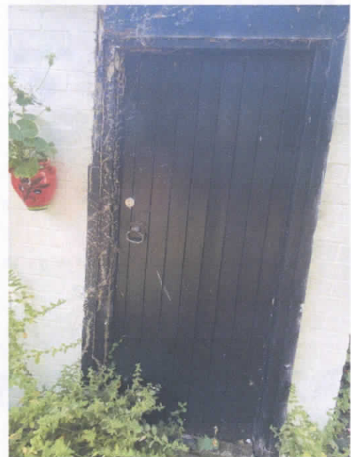
Photo 17: shed, N door on E side
