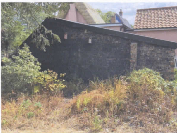
Photo 18: garage, N side
