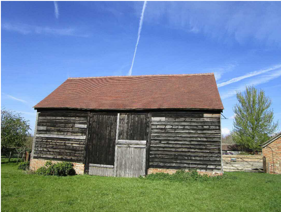
Figure 2 – The South Barn (rear elevation)
