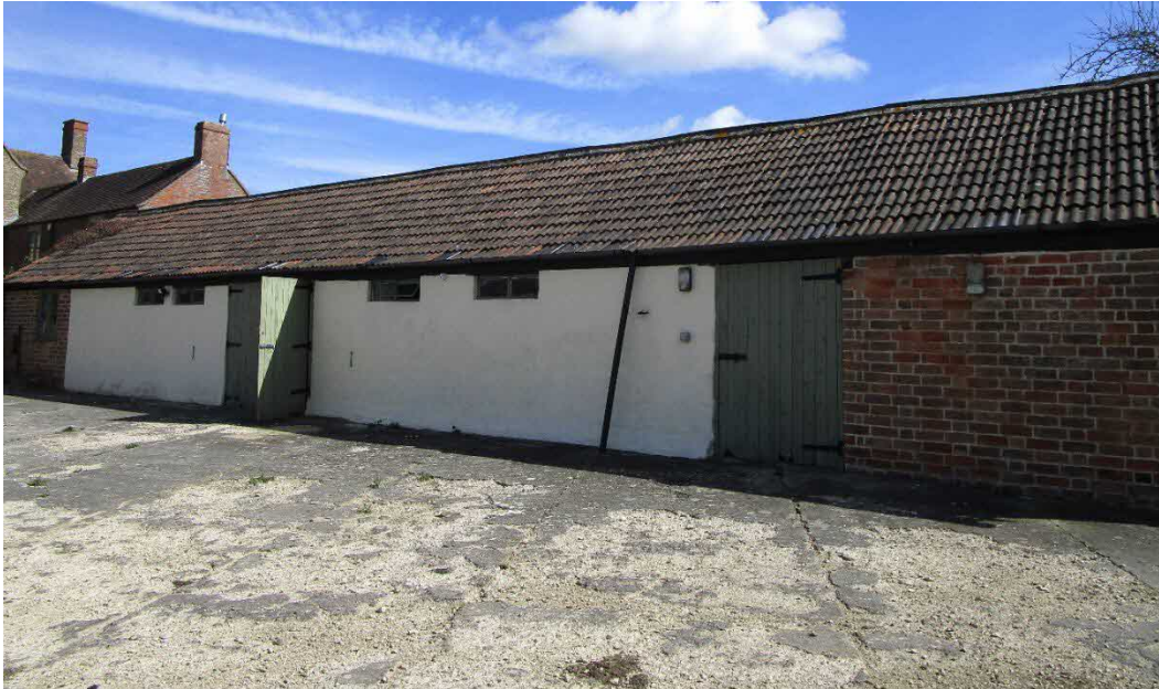
Figure 5 – External view of the East Barn
