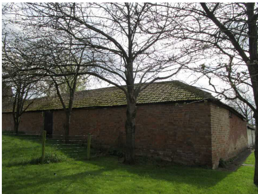
Figure 13 – the area to the rear of North Barn
