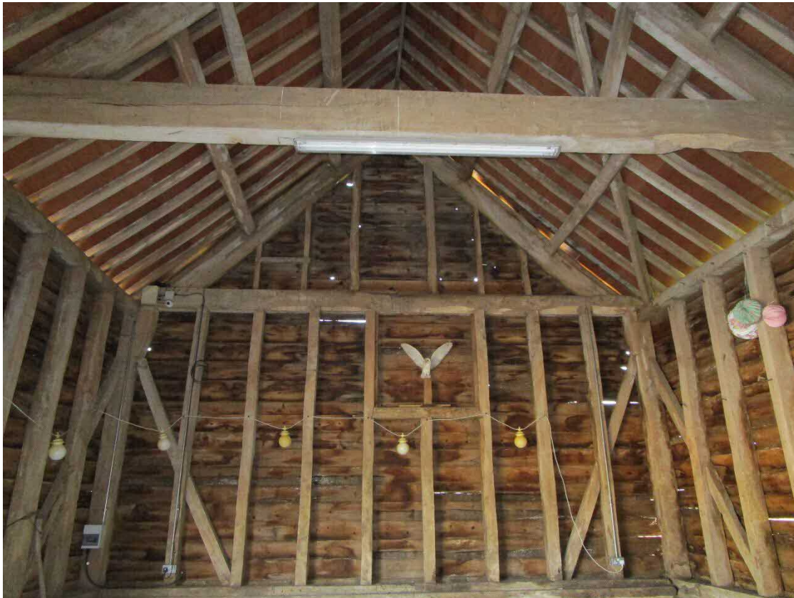
Figure 4- internal view of the south Barn
