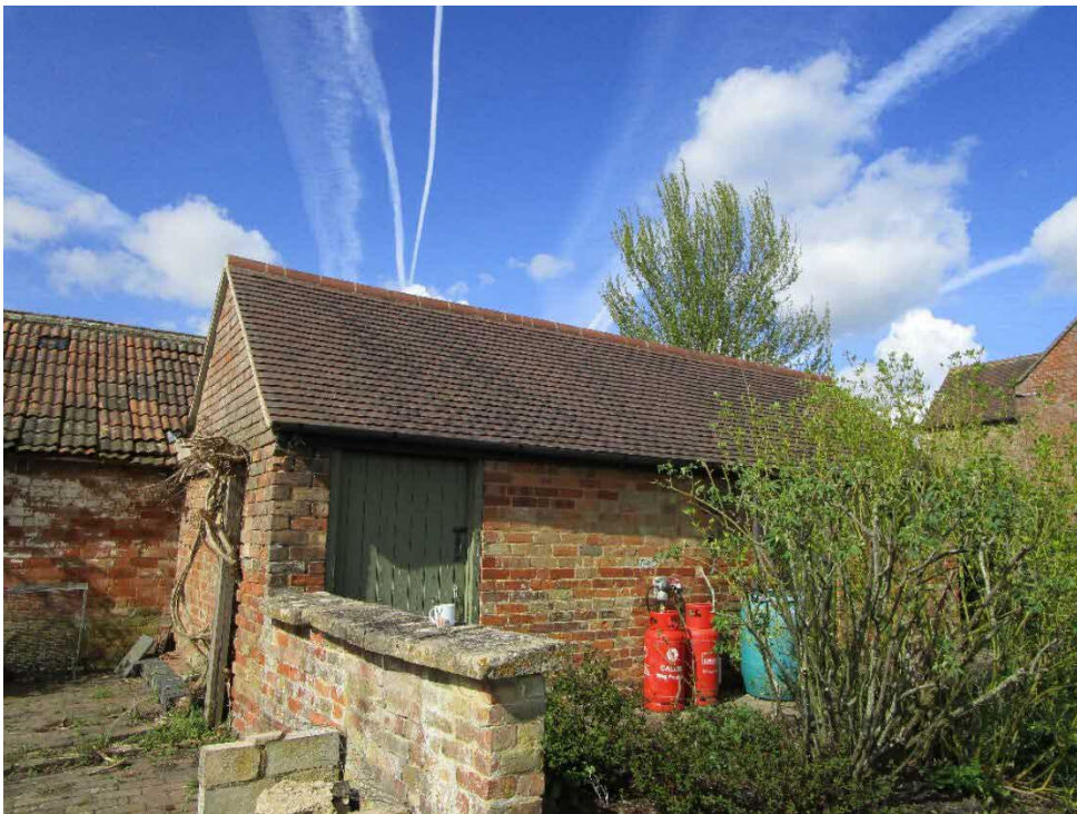
Figure 6– External view of the building adjacent to the East Barn
