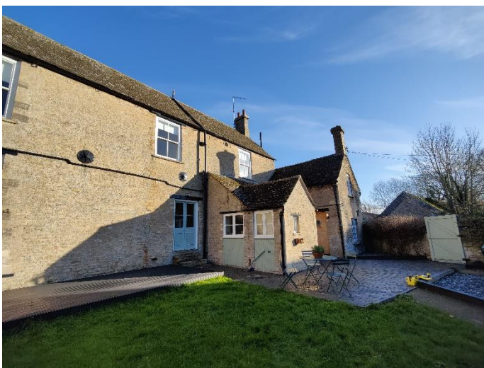
Pic 9 – rear view showing door to be reinstated
