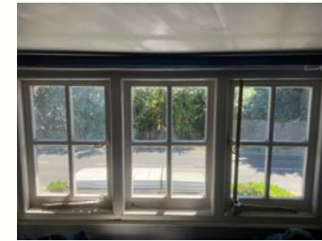
1500mm w x 750mm h Existing casement windows
