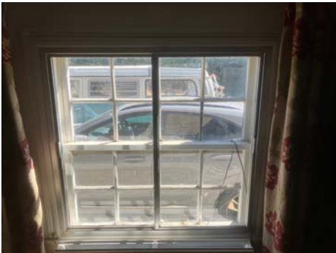
2 no 1200mm w x 1150mm h Existing 'sash' windows
