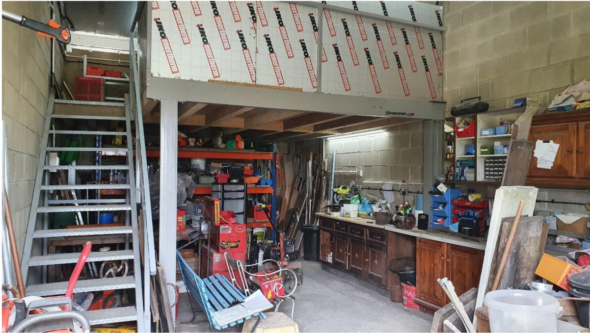
Photograph 3. Central cell mezzanine floor
