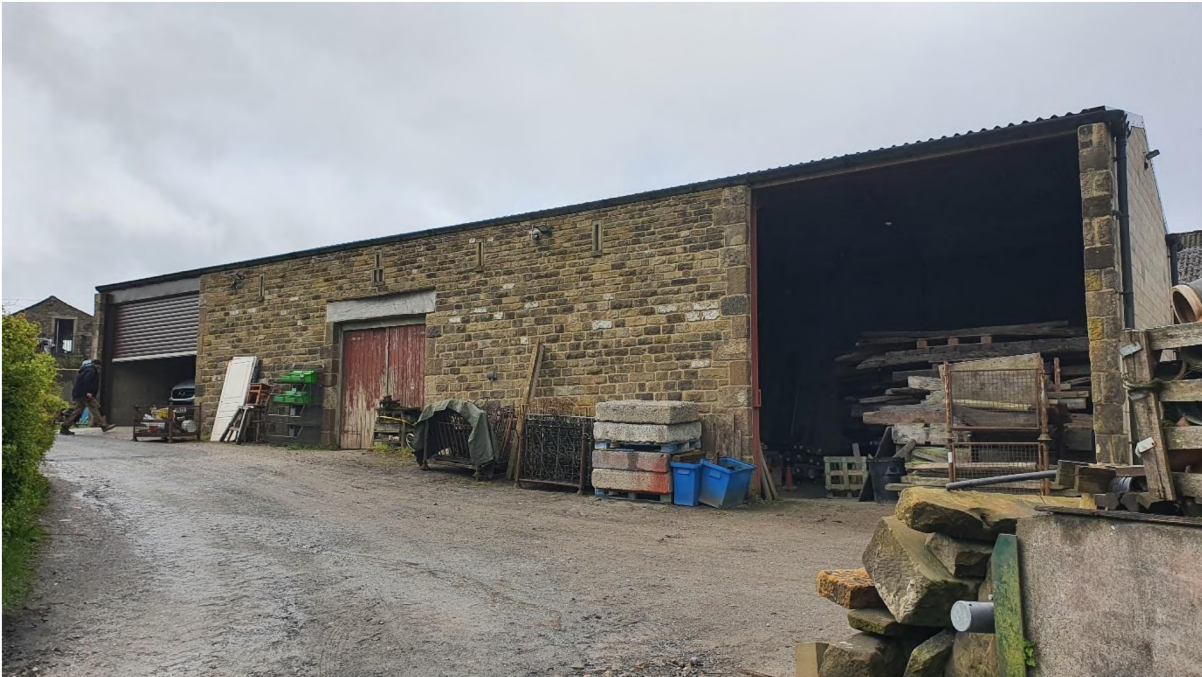
Photograph 1. General view of north east elevation
