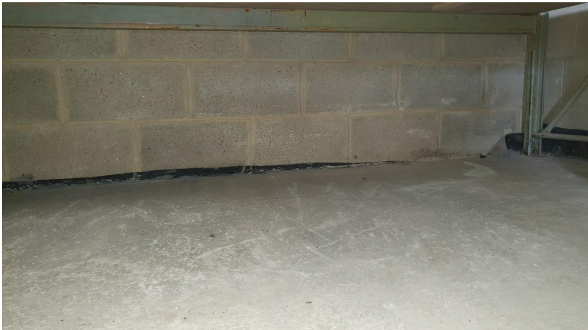
Photograph 4. Slab damp proof membrane
