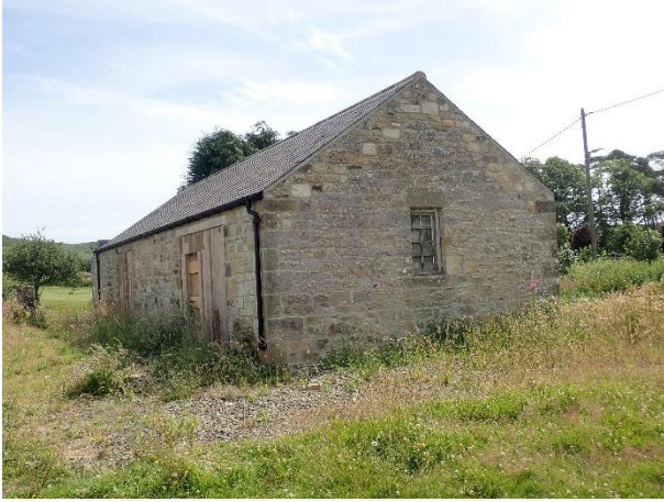
Building from the northeast
