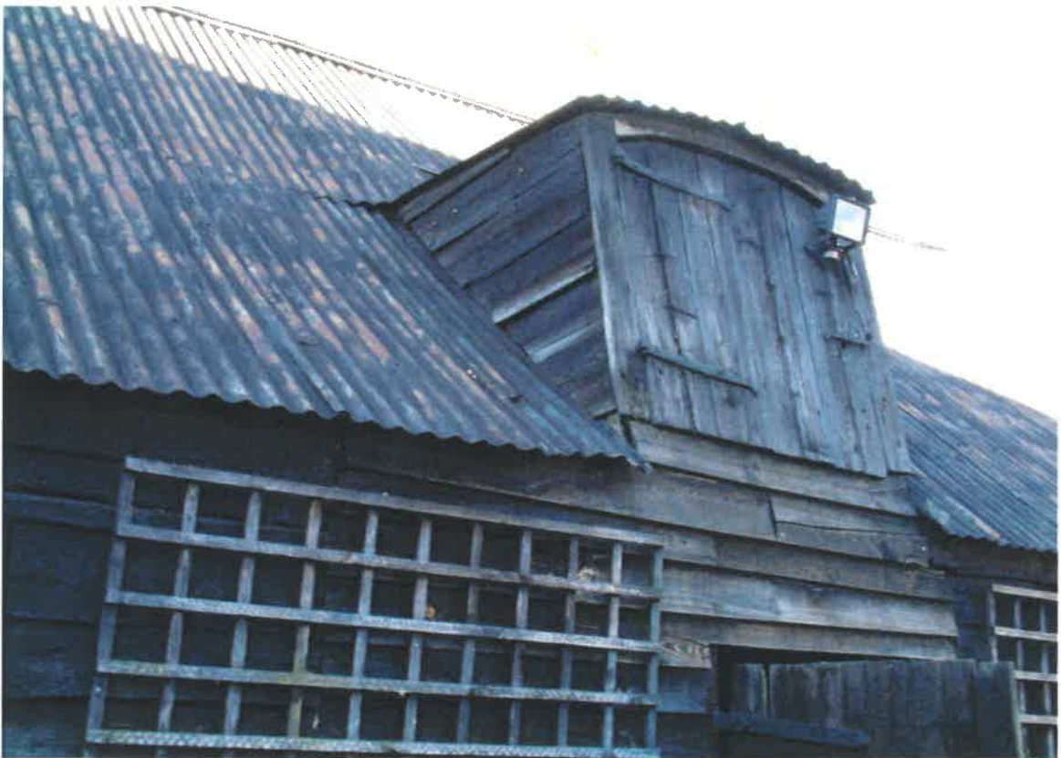
The hayloft has sunk backwards into the roof. This is not an optical illusion.
