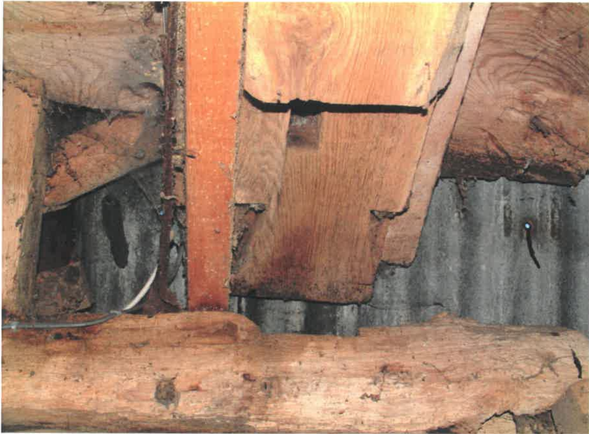
Detached dovetail from the inserted floor. Empty mortise for a tenon from its former use
