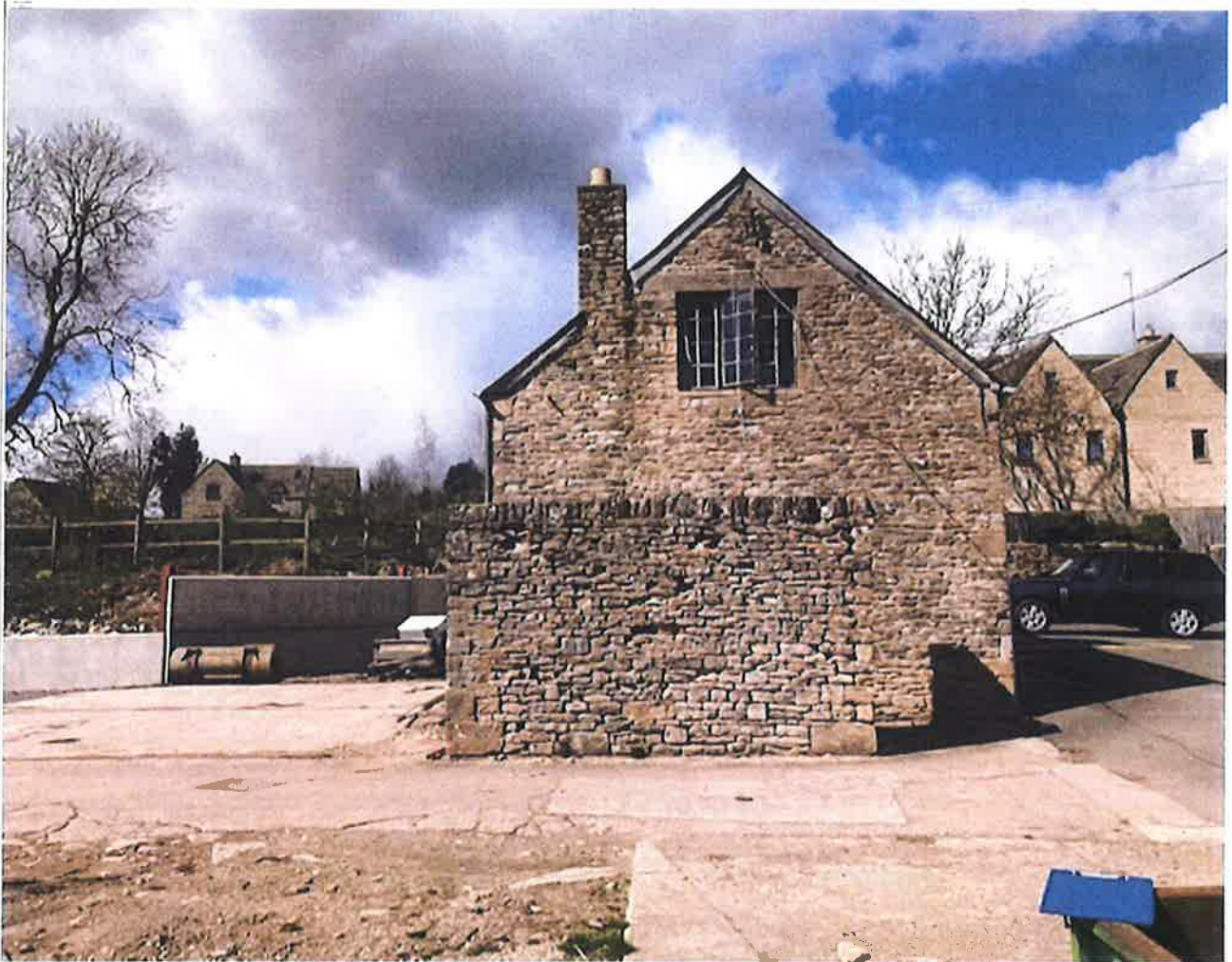
3. View of east facade of stables building showing stone gabled facade and lower screen wall to small yard; building to right behind is adjacent Audley House (see drawing 2 Block Plans for context); Note: Proposal to raise height of yard wall with new flat roof to form ground floor utility and first floor terrace to living space with conversion of window into glazed timber framed doors for access to steel balustraded terrace
