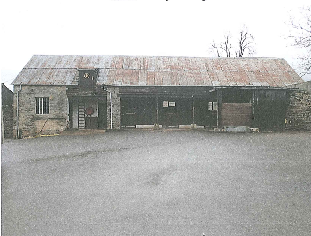
Photo 1 The surveyed building
