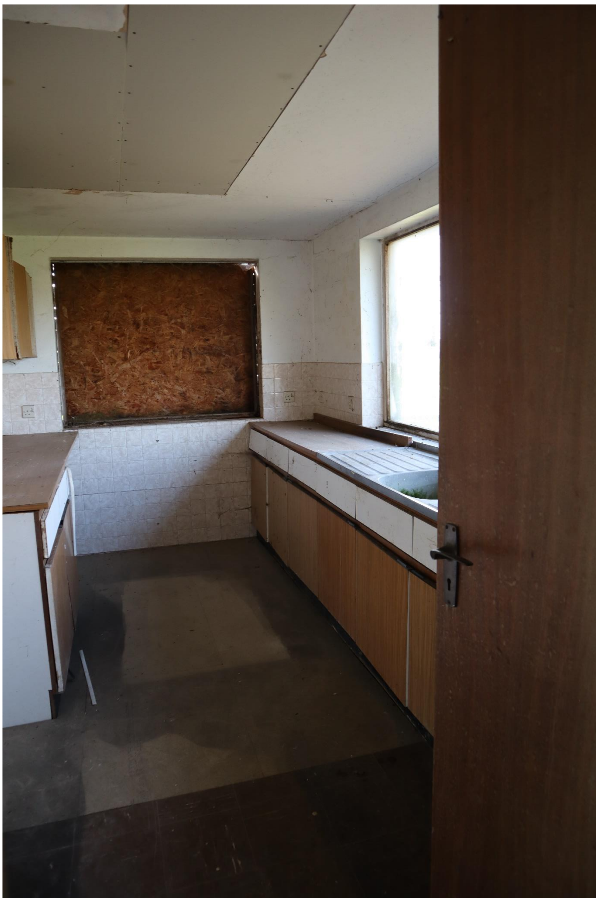
Figure 20 - existing kitchen in annexe.
