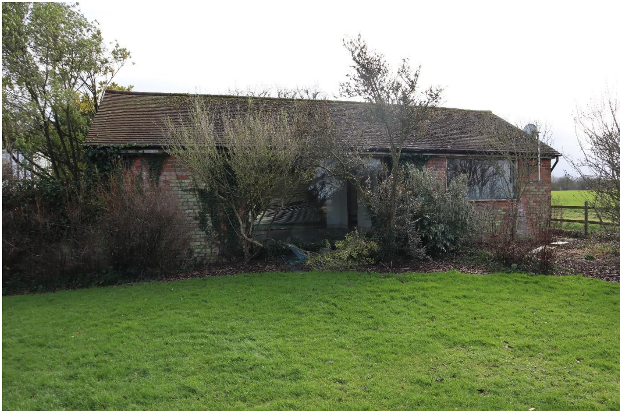
Figure 26 - north elevation of annexe.
