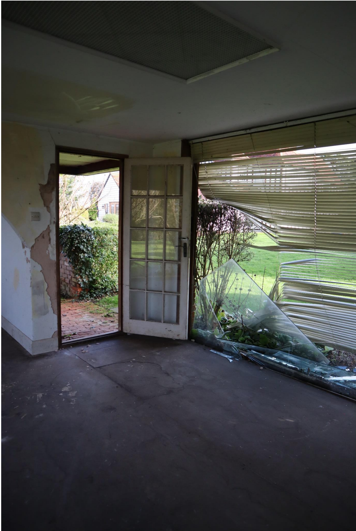
Figure 21 - main entrance into annexe, facing the main house garden.
