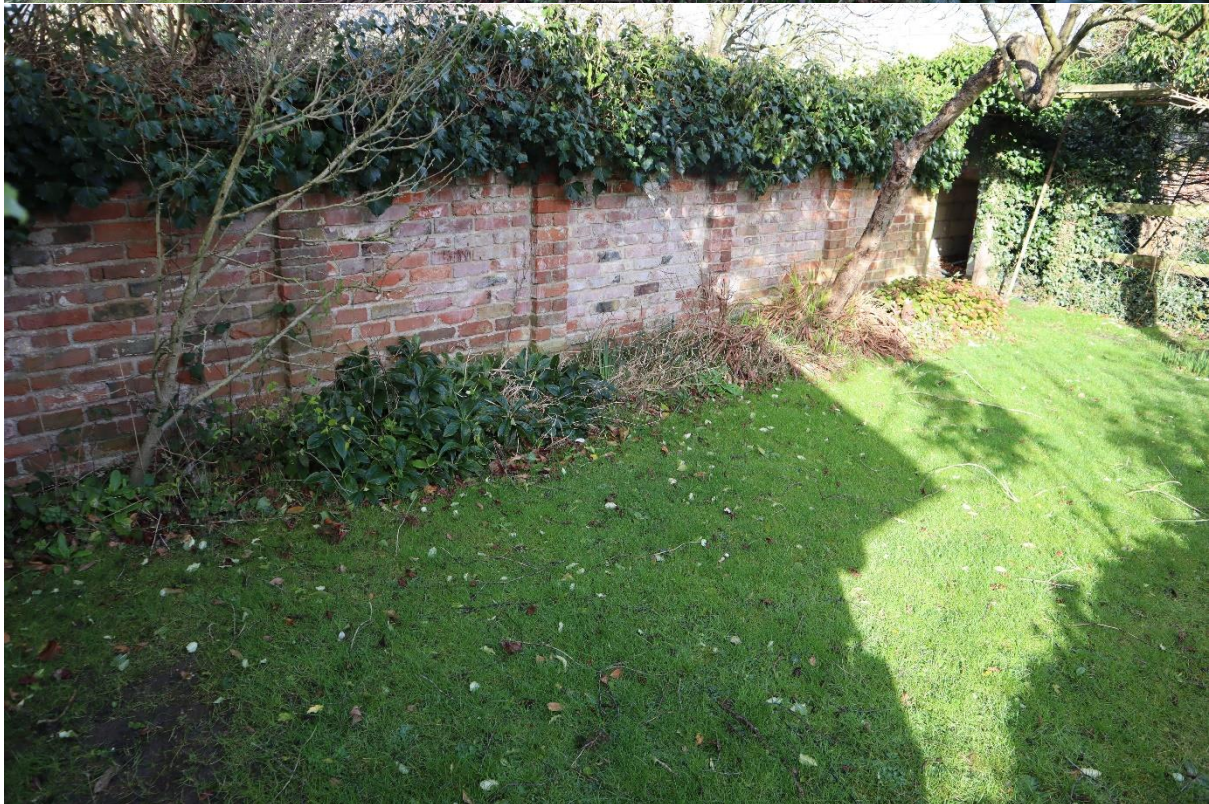
Figure 24 - former outbuilding, now walls.
