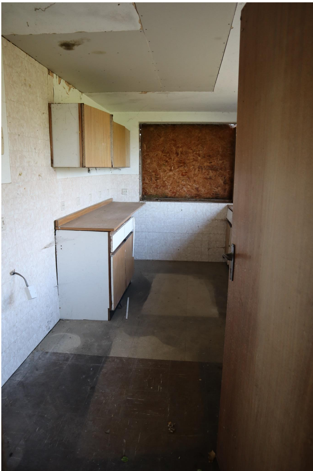
Figure 19 - existing kitchen in annexe.
