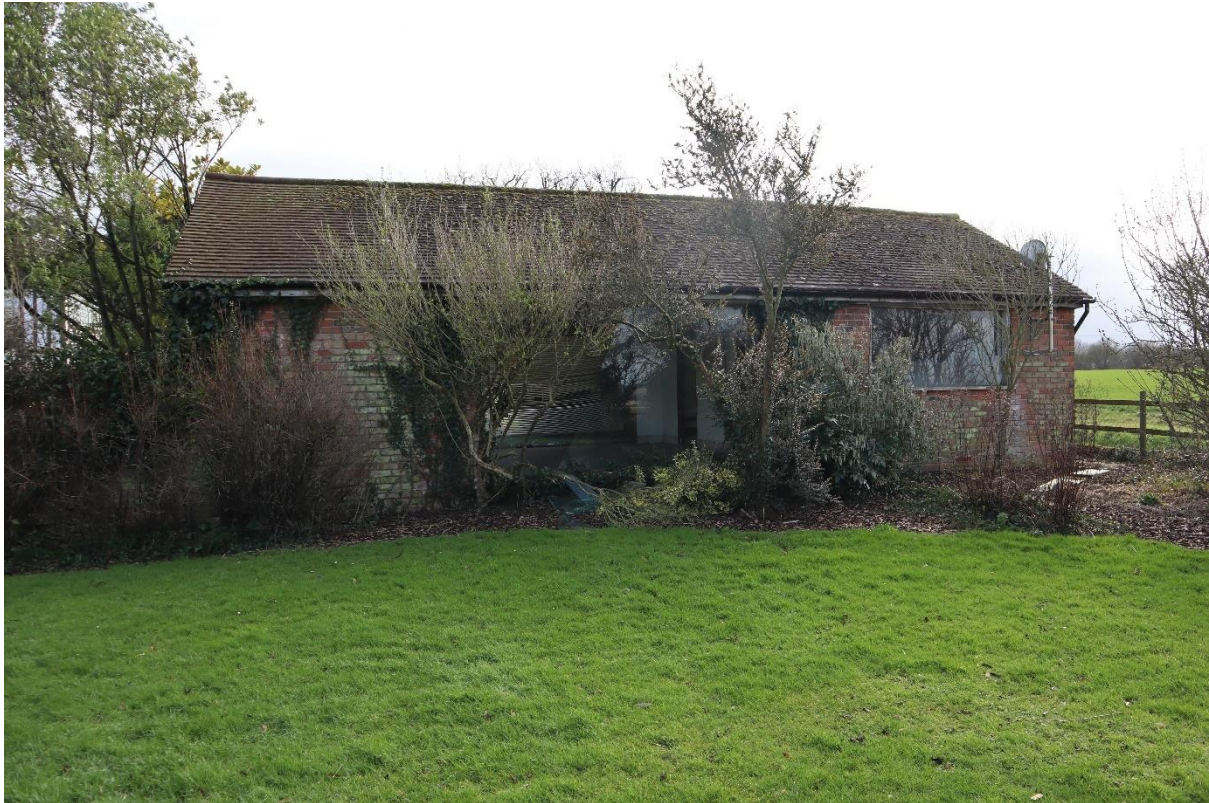
Figure 25 – rebuilt outbuilding to the north-east of the main house.
