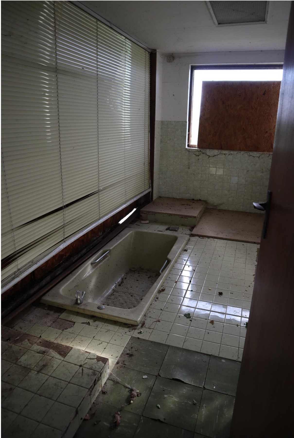
Figure 22 - existing bathroom in annexe.
