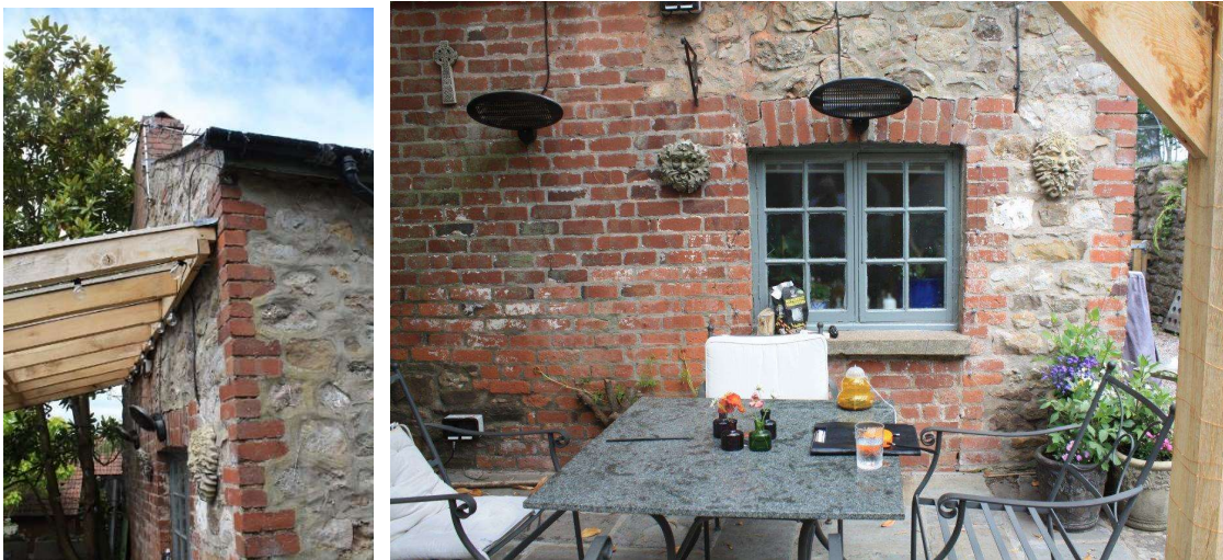
South Elevation of Tump Farm Cottage showing the chimney stack
